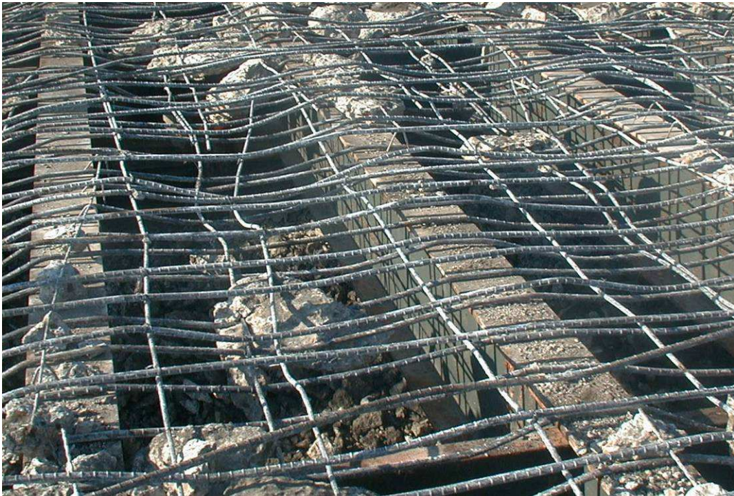
Figure 4.17. Exposed Top Flanges After MCB Deck Demolition.
