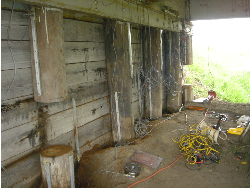
Figure 8.22. Photograph Showing Sections of Piles 3 and 7 Removed from HCB.
