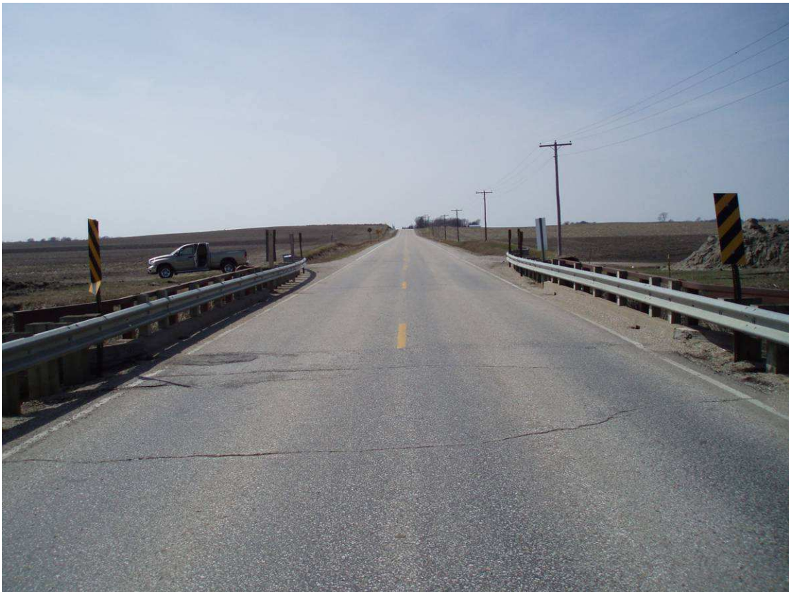
Figure 8.1. HCB Alignment View Looking West.
