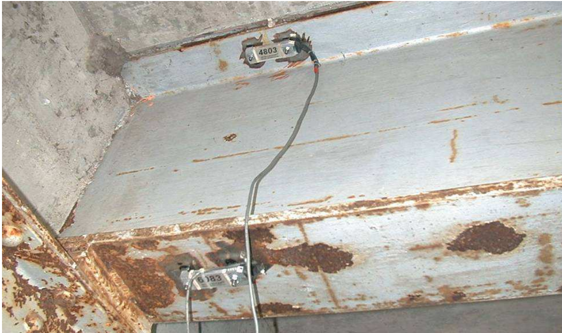
Figure 3.12. Instrumentation Near Abutment of BCB
