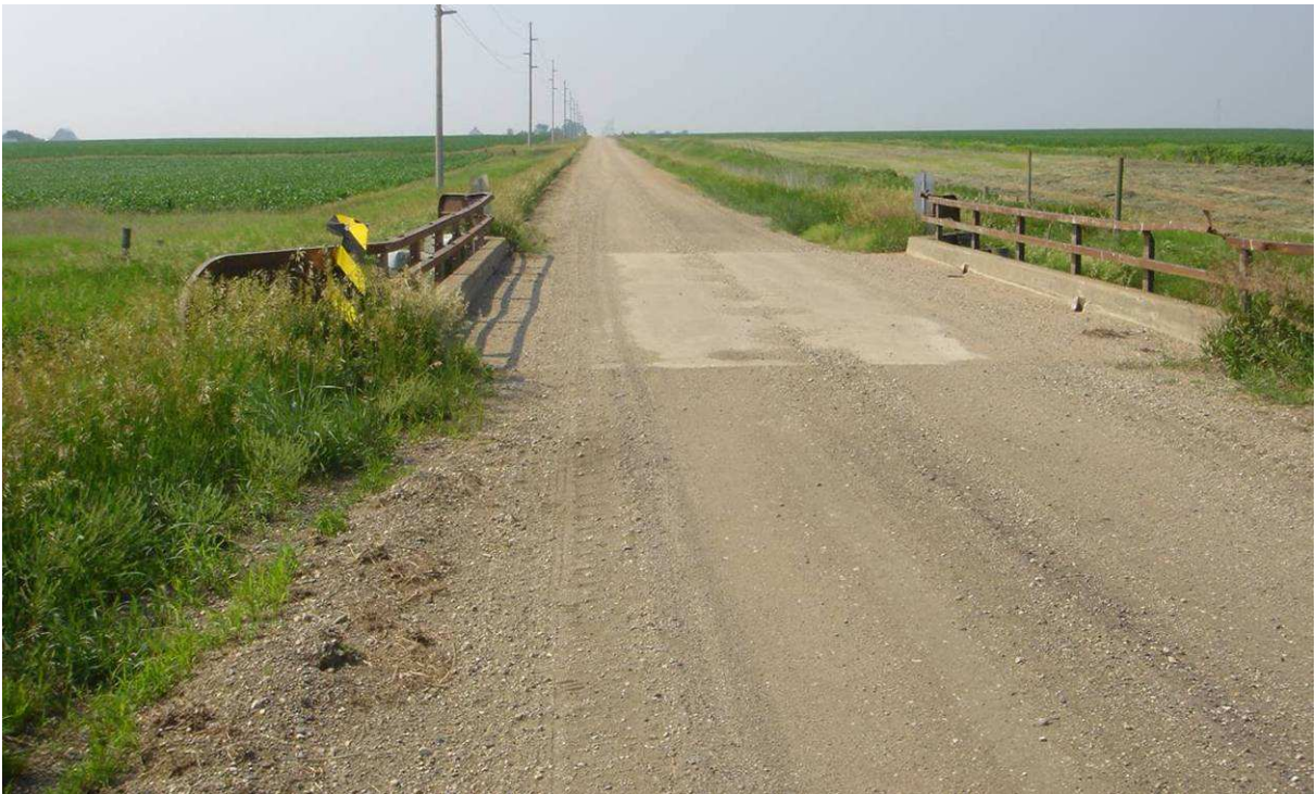
Figure 3.1. BCB Alignment View Looking South.
