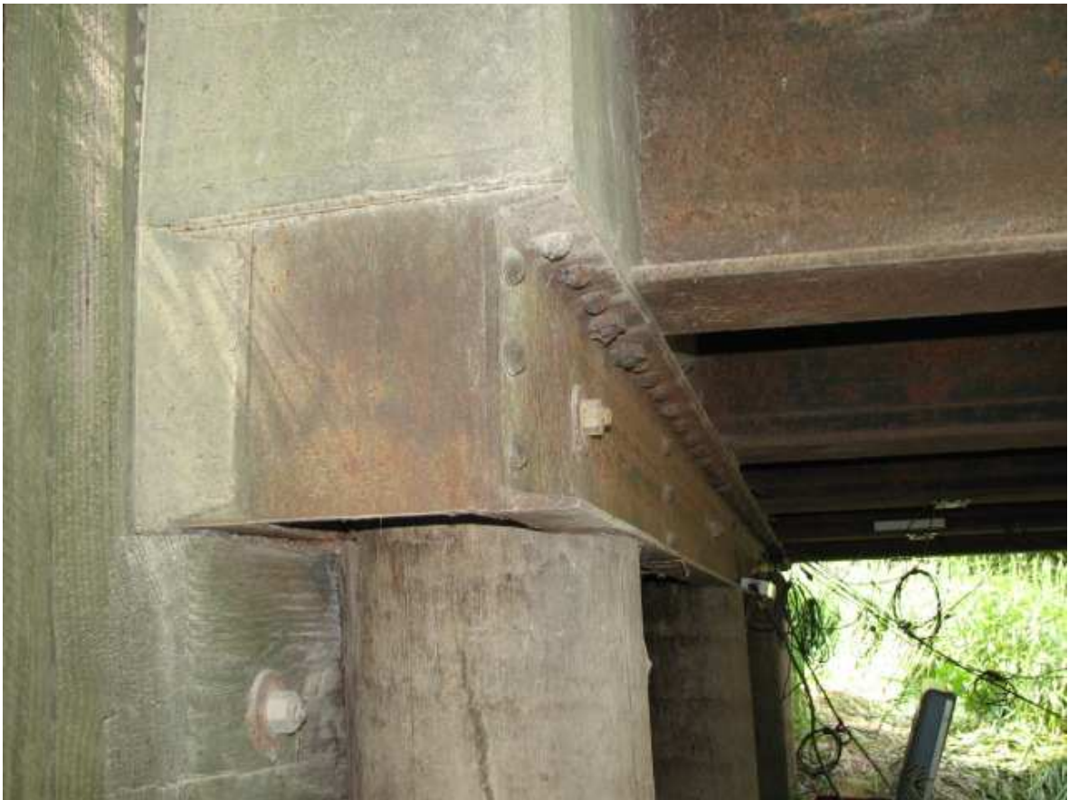
Figure 3.2. Typical Pile Cap Configuration.
