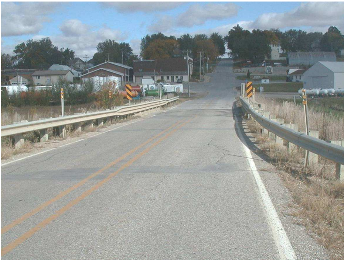
Figure 6.1. CCB Alignment View Looking North.
