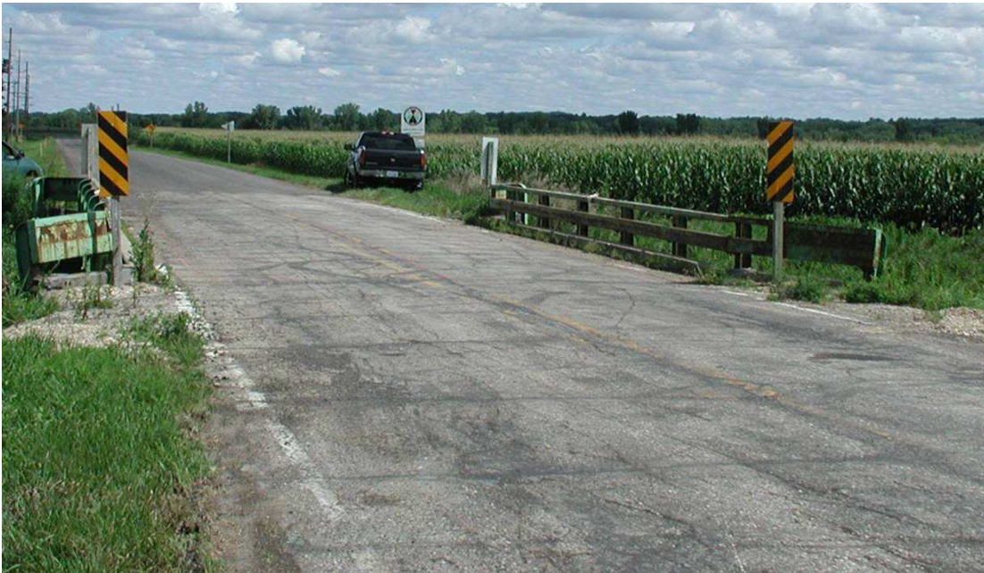
Figure 4.1. MCB Alignment View Looking North.
