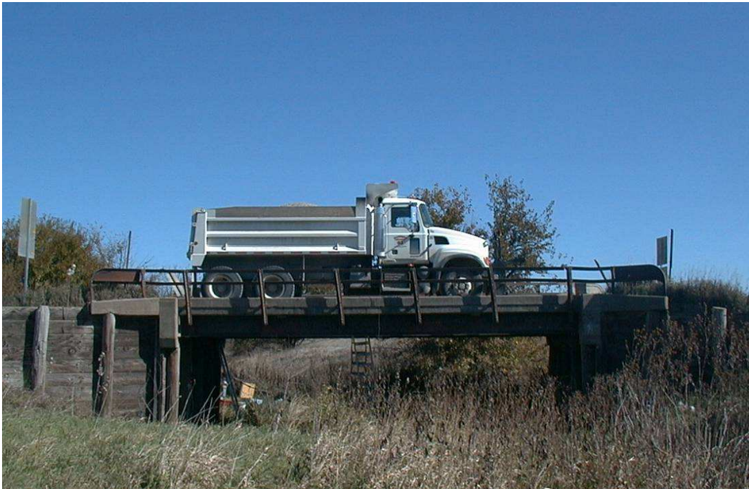
Figure 5.5. KCB1 Test Truck.
