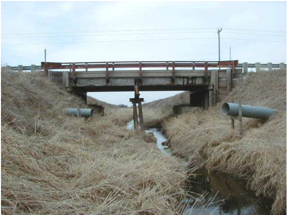
Figure 8.2. HCB Elevation View of Bridge Looking North.
