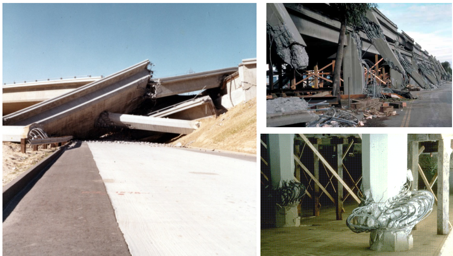
Figure 1-2: Earthquake damage: San Fernando (left); Loma Prieta (top right); Northridge (bottom right) [photos accessed through USGS website (2009)]
