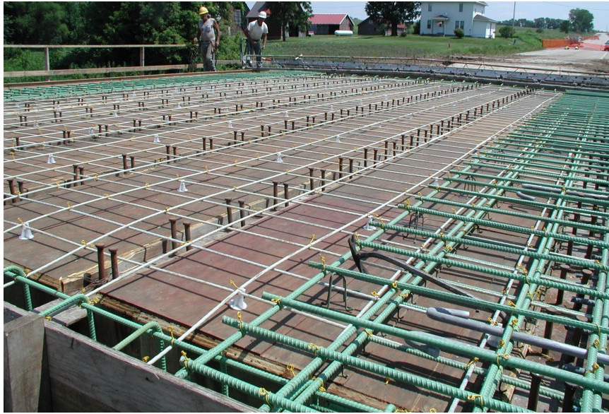
Figure 2.4. Epoxy coated steel and GFRP reinforcement.
