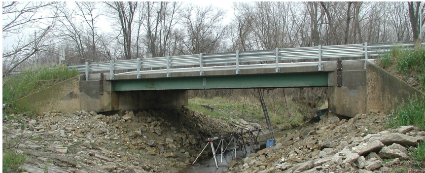
Figure 2.5. Elevation of Tama County SFD bridge.
