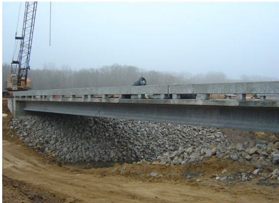
Figure 3.4. Elevation of Wapello County UHPC bridge.
