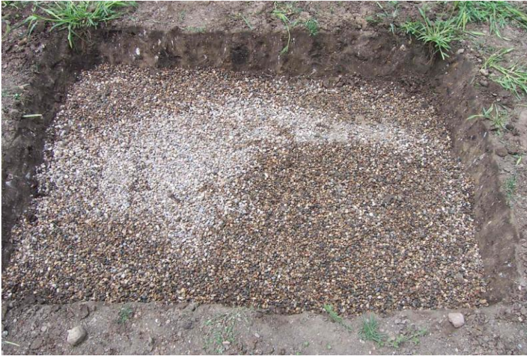
Figure 47. Aggregate base at test location
