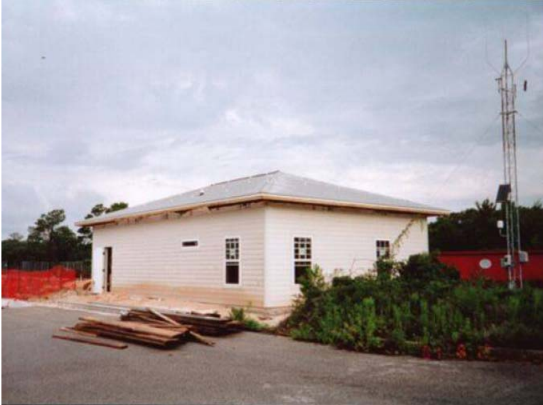
Figure 6.1. Low-rise field test structure constructed in Pensacola, Florida (FPL, 2006)
