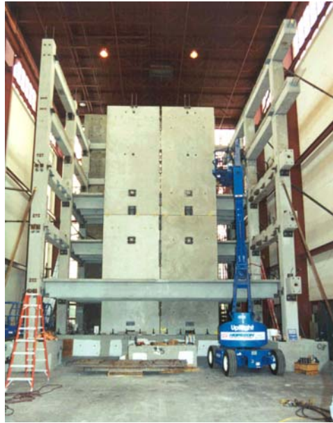
Figure 4.4. The PRESSS test building after erecting the jointed wall system
