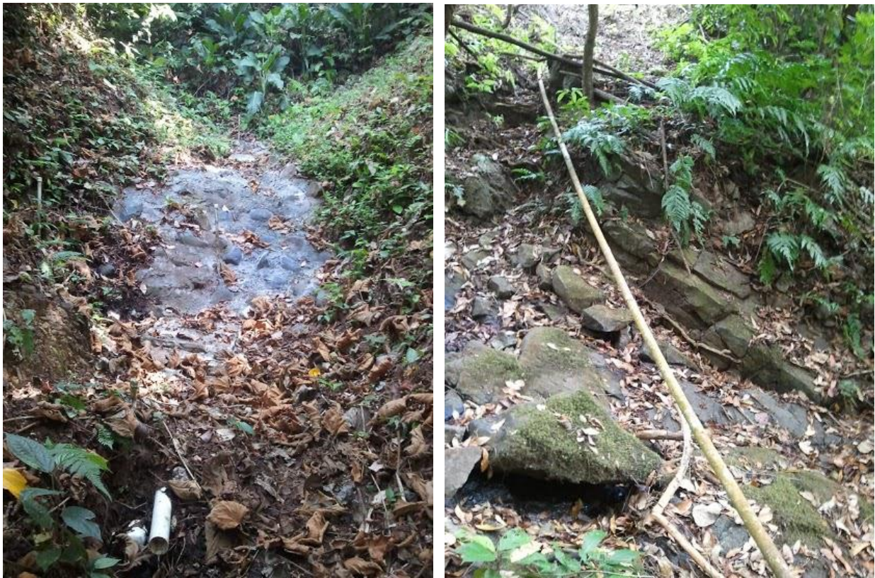
Figure 5: Spring Source (left) and Distribution Line (right) of the Water System
