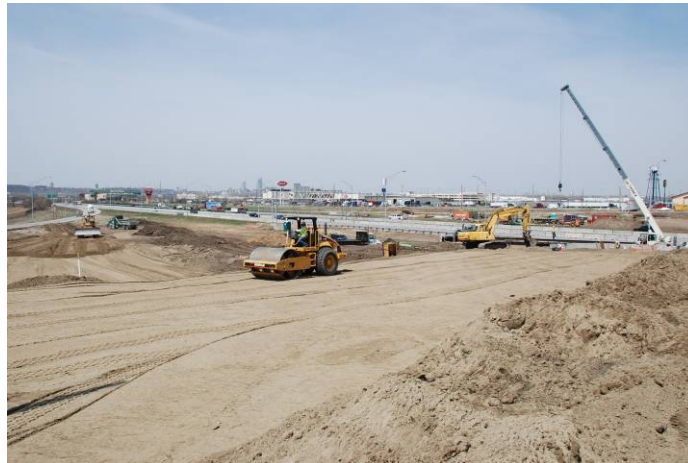
Figure 5. The location of the new bridge during stage 1 (Photo to the west of existing bridge)
