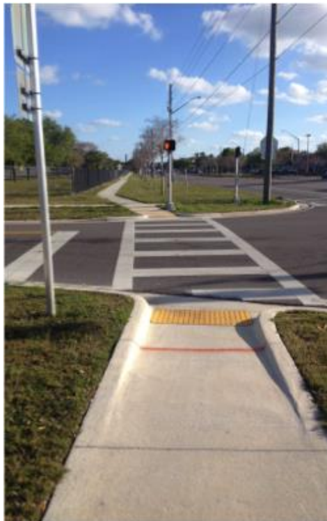
Figure 3 High visibility crosswalk
