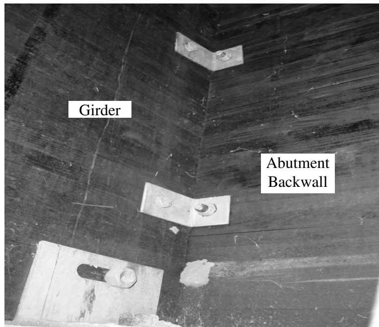
Figure 4. Girder to abutment backwall connection
