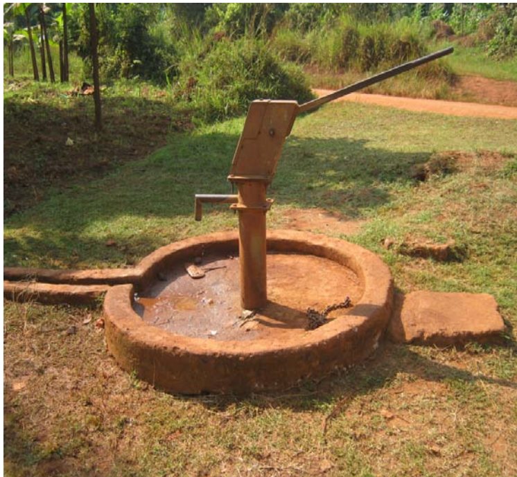
Figure 15: Borehole that consists of groundwater extraction by manual pumping (Photo: C. Prouty)
