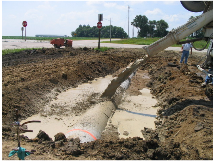
Figure 5.13: Pouring the flowable mortar
