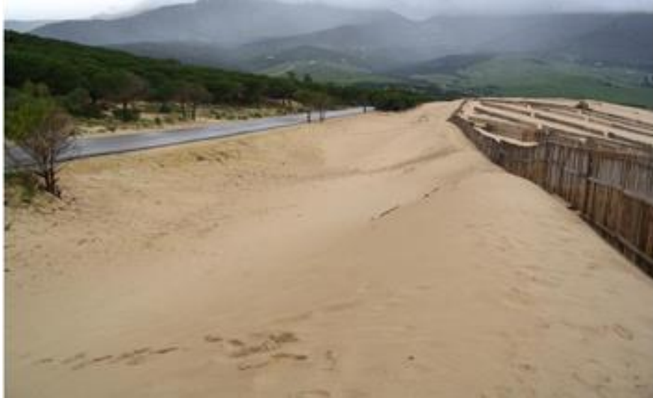
Figure 1.7 Structural sand fence installed along a highway to minimize sand drifting on the road (Source: http://members.virtualtourist.com/m/p/m/1ed4e5/ ).
