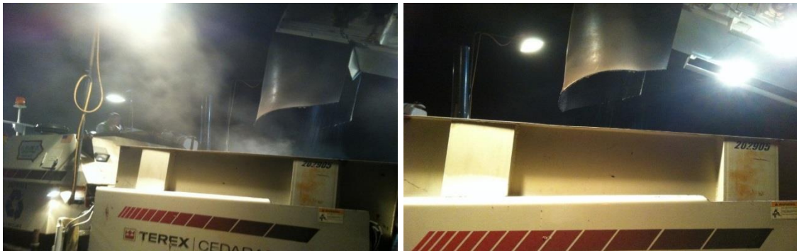
Figure 5.3 HMA (left), and WMA (right) Emissions during Construction.
