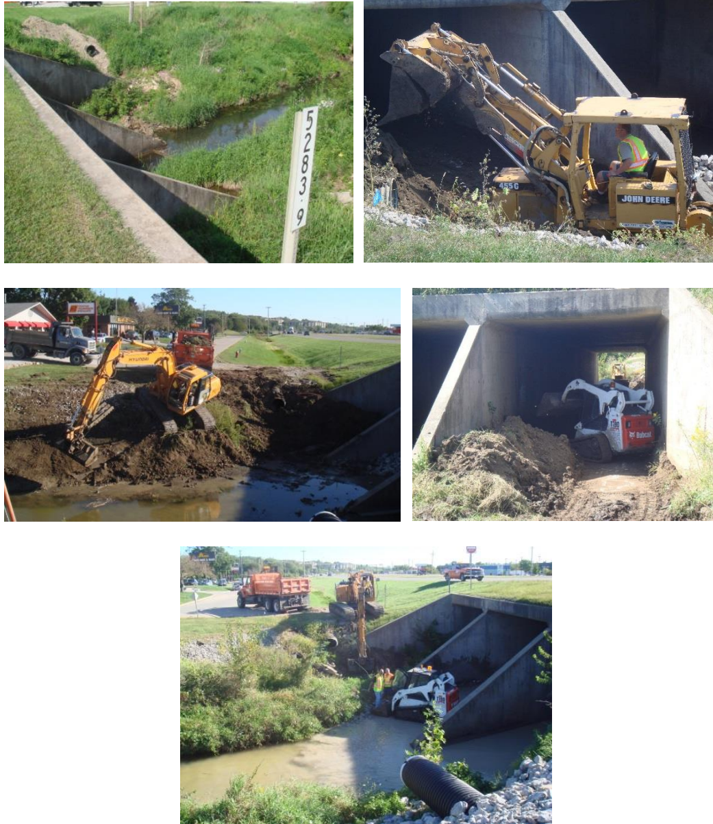
Figure 2.8 Culvert sediment cleaning involve excavator (Muste, 2014)
