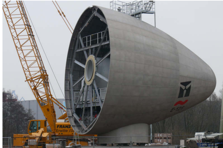
Figure 2-7: Enercon E-126 nacelle [33]
