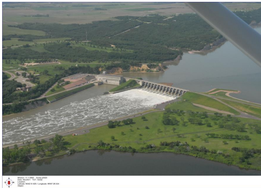
Figure 1.3: Missouri River, Gavins Point Dam and Reservoir (Tretbar, 2011)
