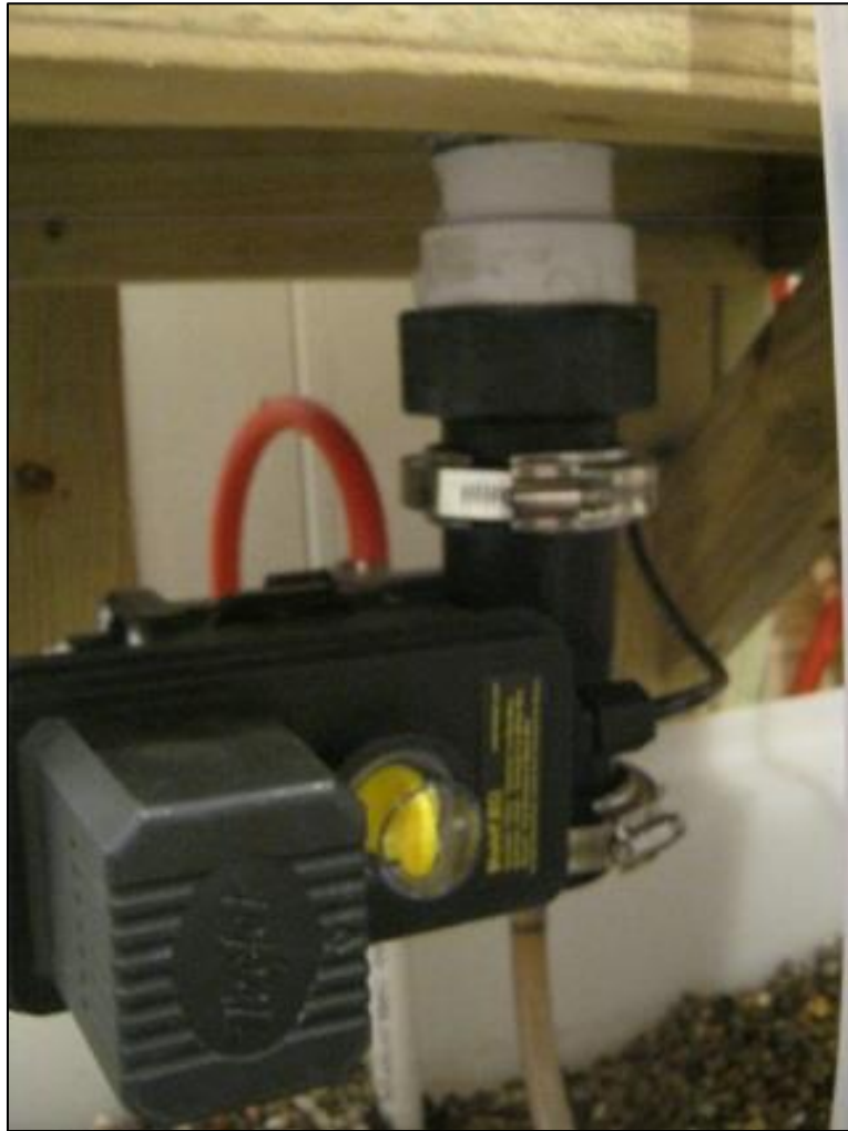
Figure A4. An image of an electronic dose valve placed directly under a dose tank.
