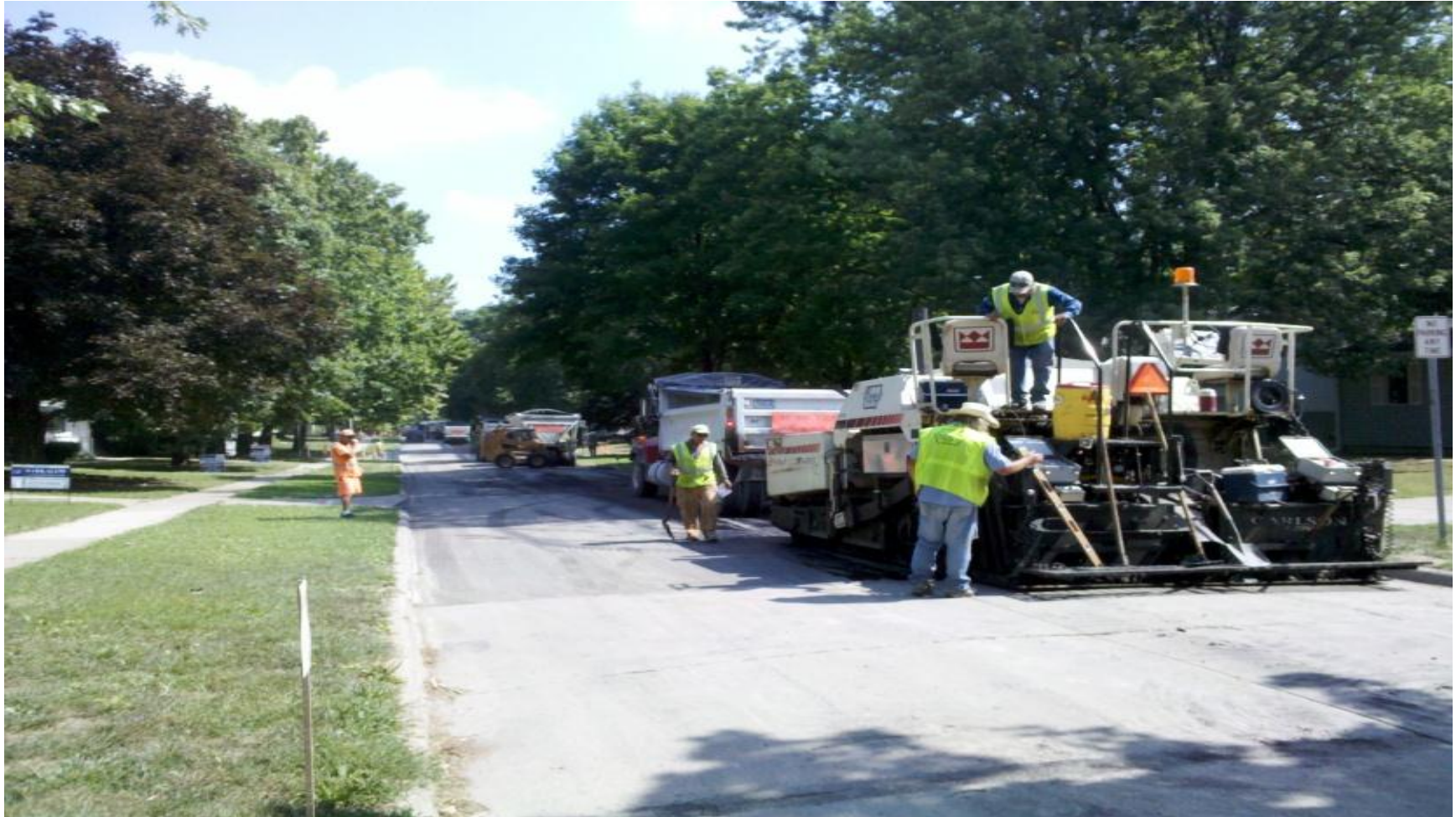
Figure 4.10: Miami Drive job site
