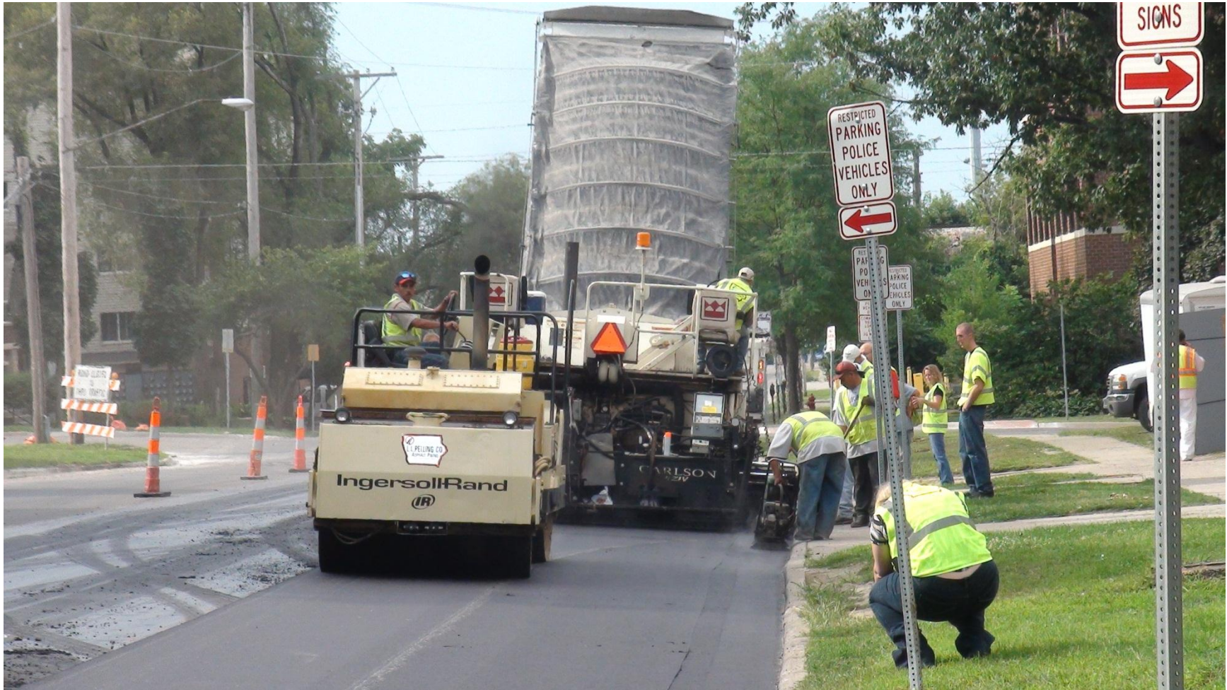
Figure 4.9: Capitol Street job site
