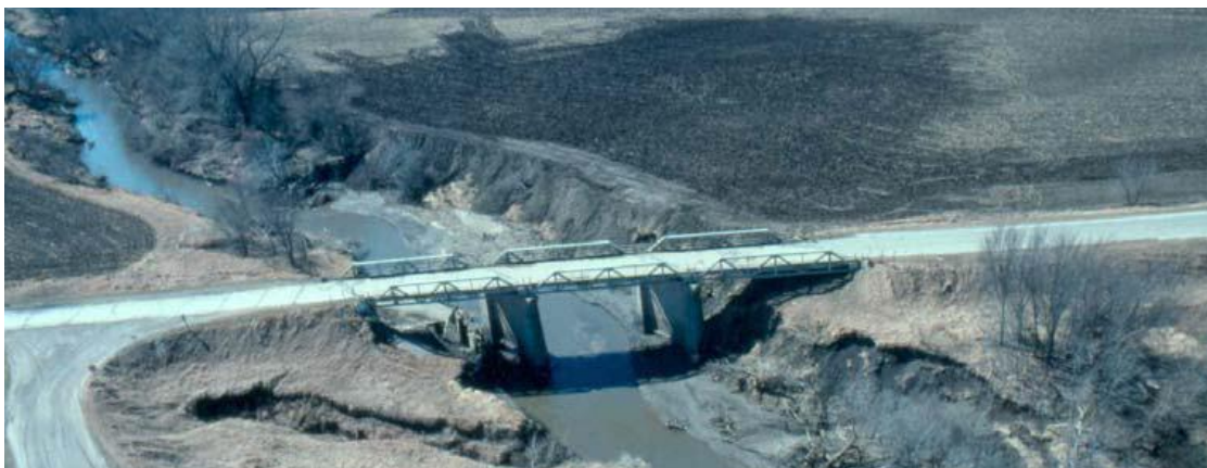
Figure 1-1 The Willow Creek bridge failure, where the bed elevation was lowered due to erosion. Extensive erosion can expose the subsoil leading to the formation of an abrupt step in the channel bed, varying from few centimeters to many meters in depth. This abrupt step is known as a head-cut and progresses upstream putting at greater risk the structural integrity of the bridge (after Ettema et al., 2006).
