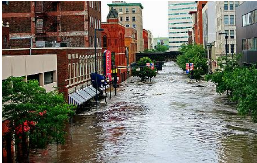
Figure 1.1: Downtown Cedar Rapids, Iowa during 2008 flood (Olson, 2008)
