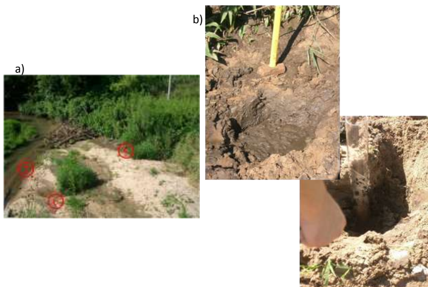
Figure 3.24 Sediment cores were collected in the sedimentation upstream the culvert shown in Figure 3.22
