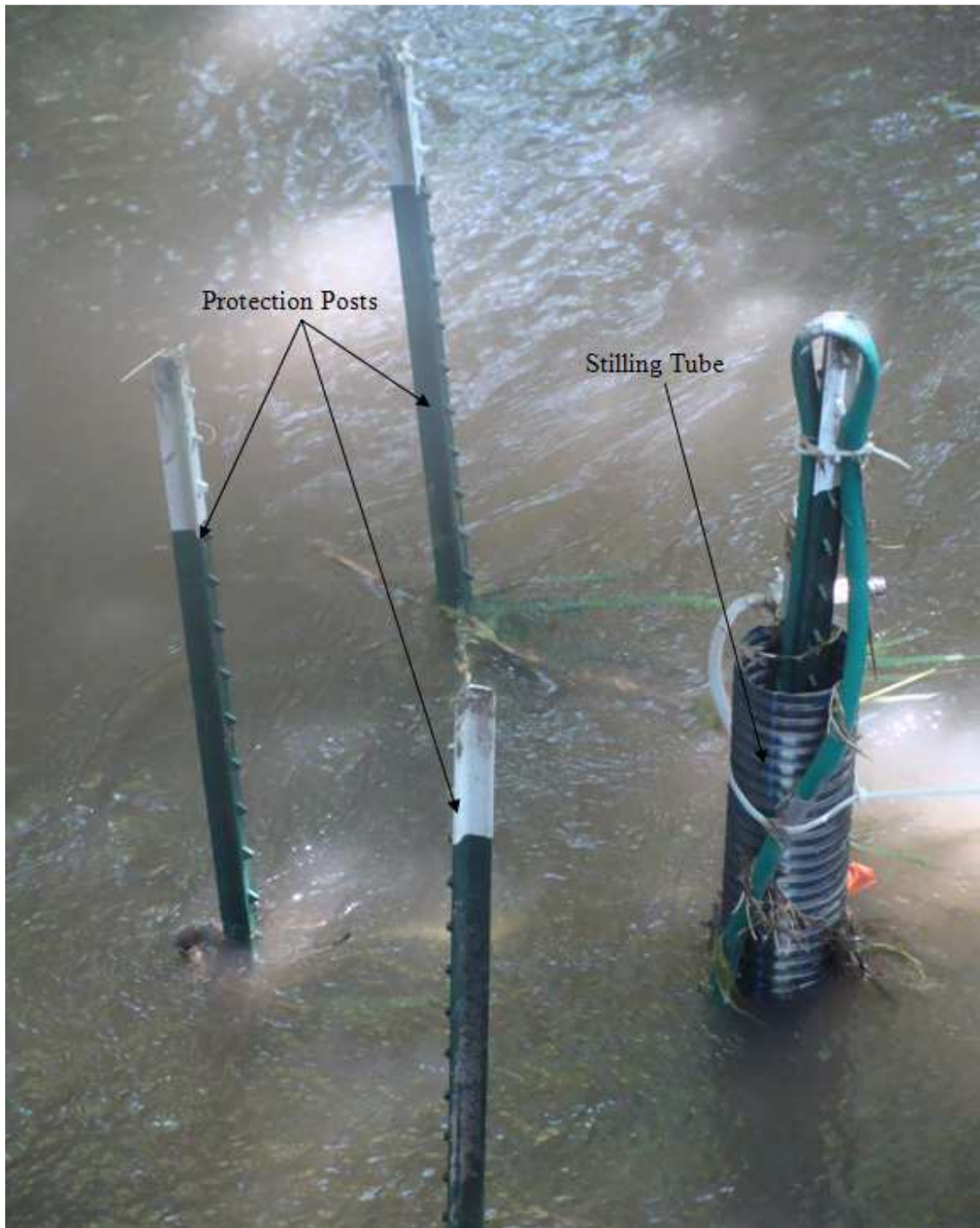
Figure 4.2. Installed pressure transducer
