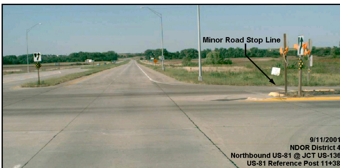
FIGURE 16. Expressway intersection where minor road stop bar could be moved forward
