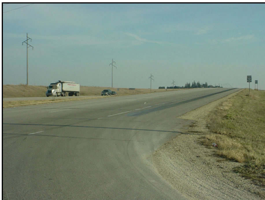
FIGURE 68. Sight distance issue for eastbound CSAH-9 traffic looking south
