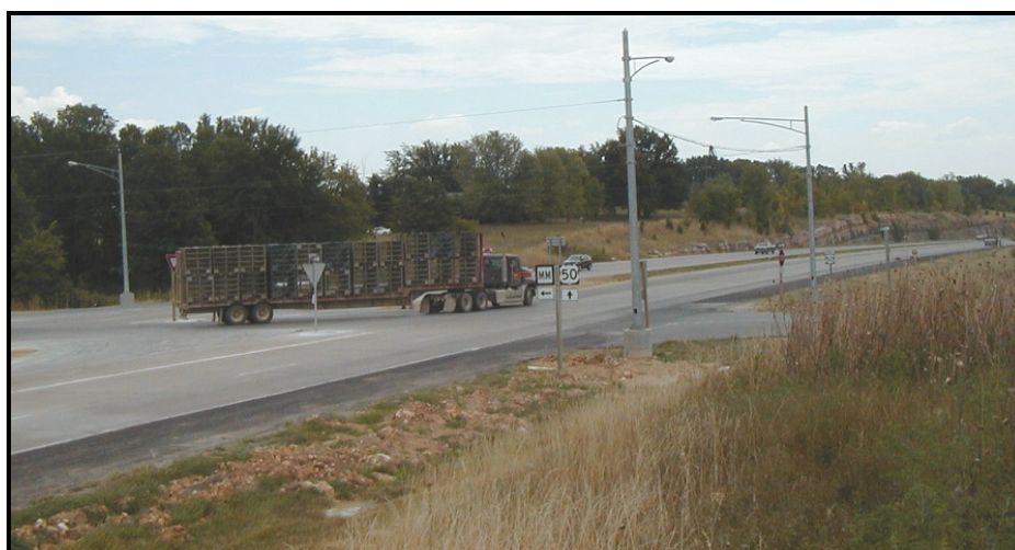
FIGURE 77. MoDOT MAL at US-50 & Route MM
