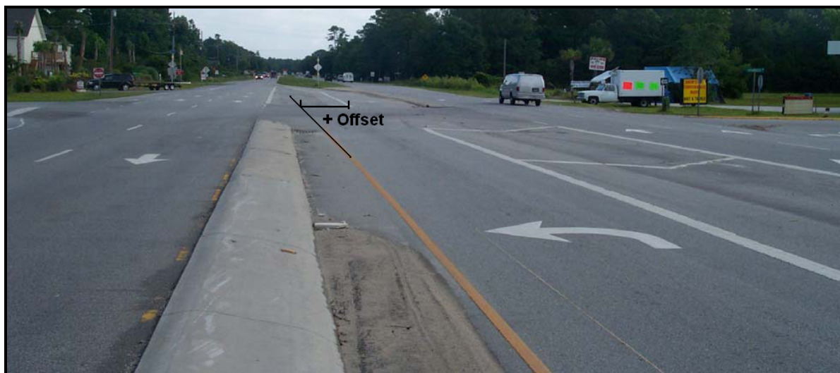
FIGURE 99. Parallel offset left-turn lanes at US-421 & SR-1576/1531 (northbound view)
