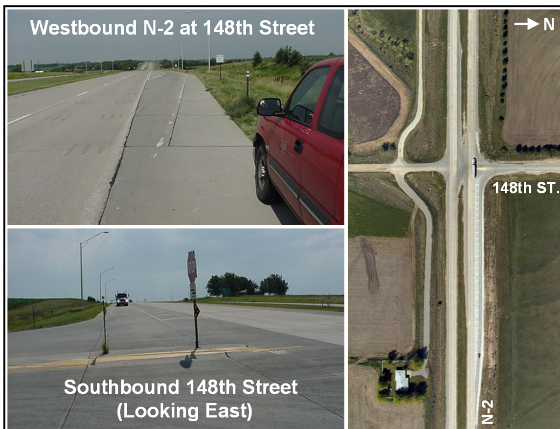
FIGURE 86. Offset right-turn lane at N-2 & 148 th Street – near Lincoln, NE
