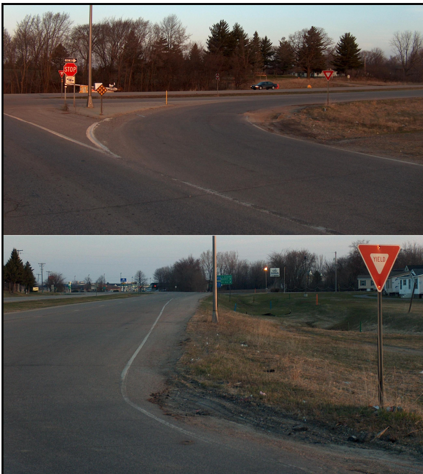
FIGURE 17. Right-turn acceleration lane in Minnesota
