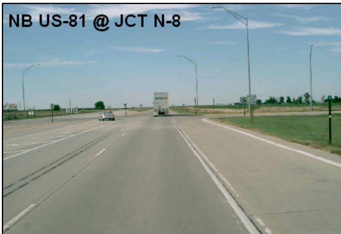
FIGURE 89. Observed misuse of offset left-turn lane in Nebraska
