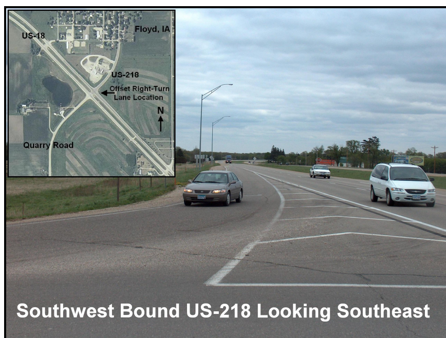
FIGURE 84. Offset right-turn lane at West Junction of US-18 & US-218 – Floyd, IA
