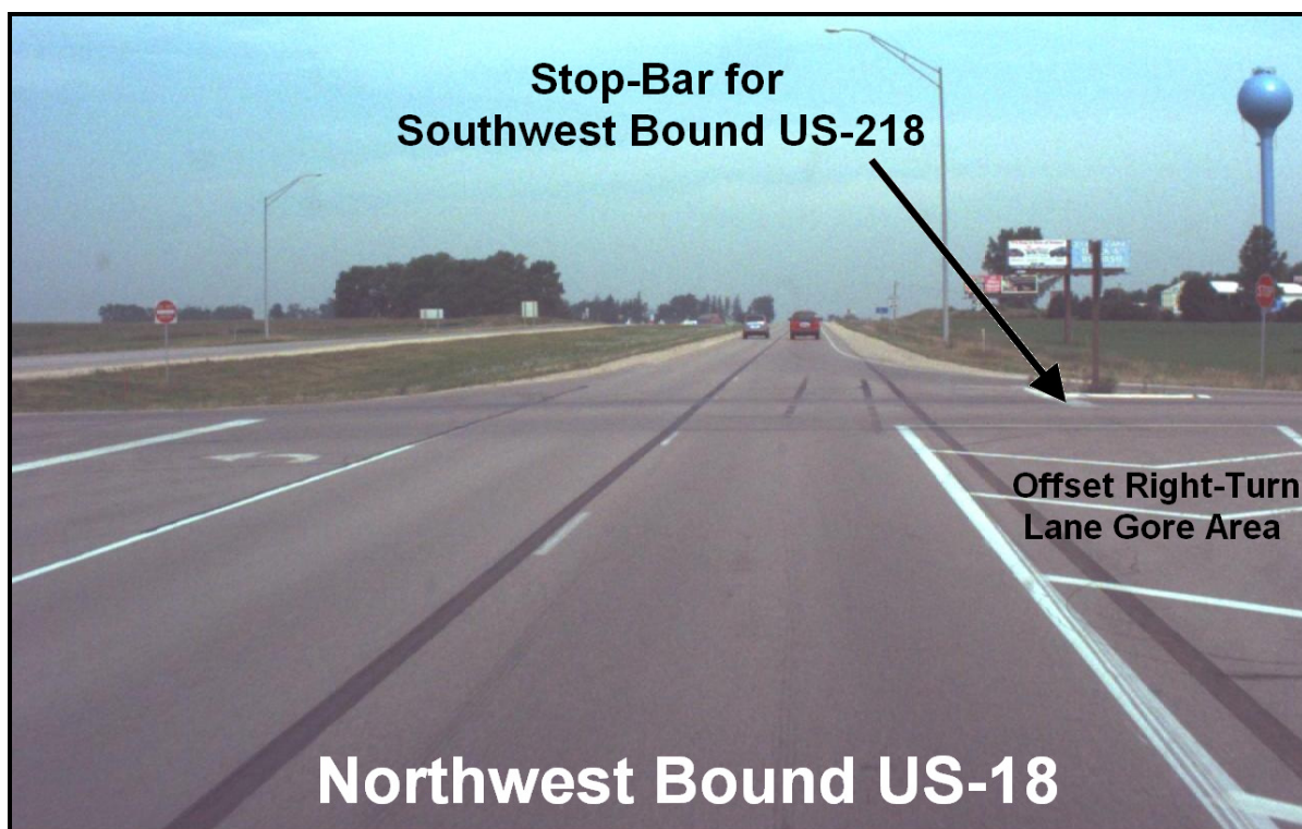
FIGURE 85. Stop bar location on southwest bound US-218
