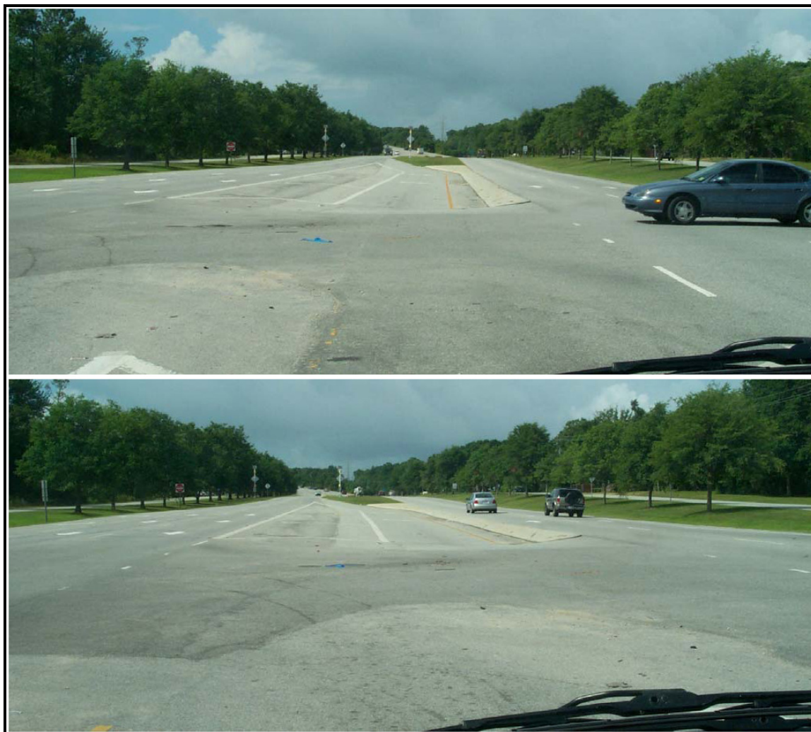
FIGURE 100. Parallel offset left-turn lanes – US-421 & SR-1576/1531 (southbound view)
