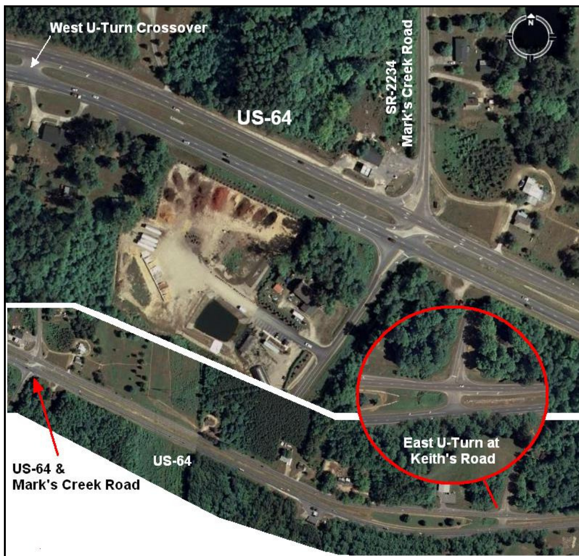
FIGURE 47. Aerial photo of J-turn intersection at US-64 & Mark's Creek Road
