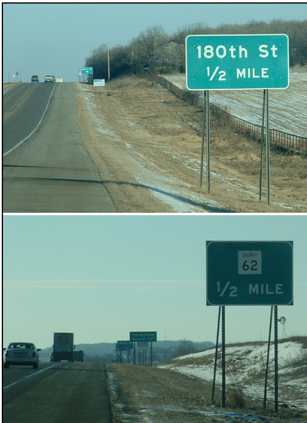
FIGURE 106. Freeway-style advance intersection guide signing along US-52
