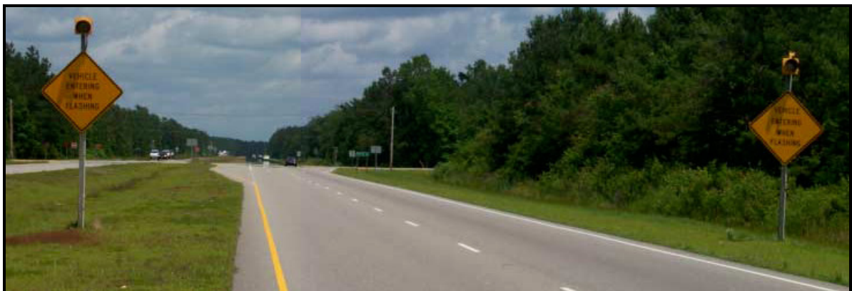
FIGURE 109. Dynamic VEFW signs on eastbound US-74/76 at SR-1800 (Blacksmith Rd)
