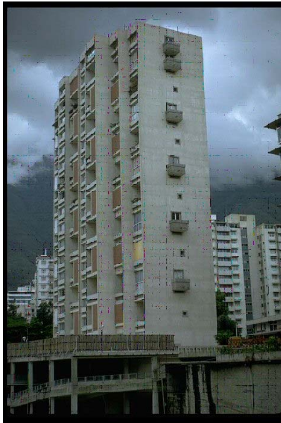
Figure 1-1: Plaza 1 Apartment Building that was undamaged during the Caracas Earthquake [1]
