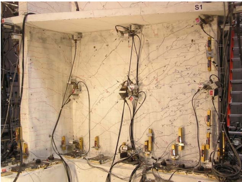
Figure 4-44: Condition of Web at First Floor After Subjected to 1% Drift Cycles
