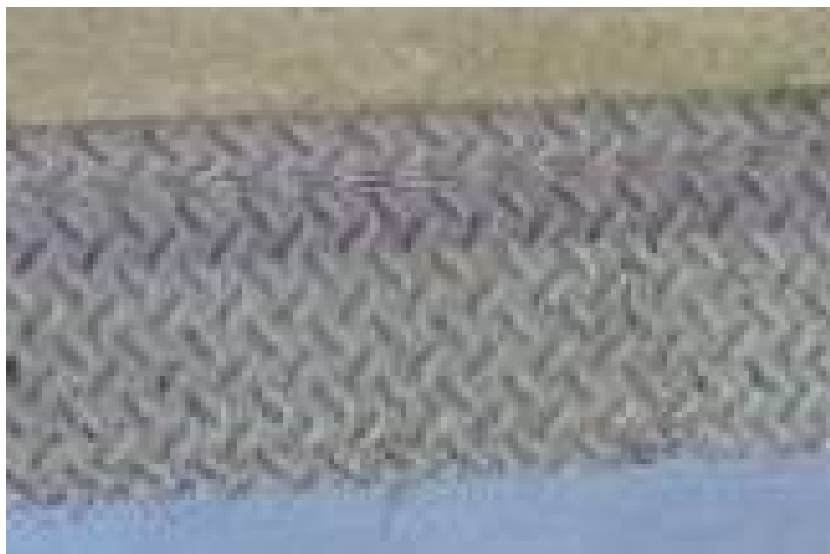
Figure 2.3. Textured surface of transverse joint.
