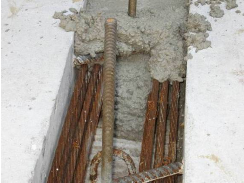
a) concrete flowing in channel
