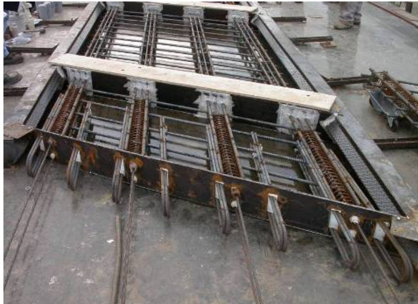
b) double hooks and prestressing strands
