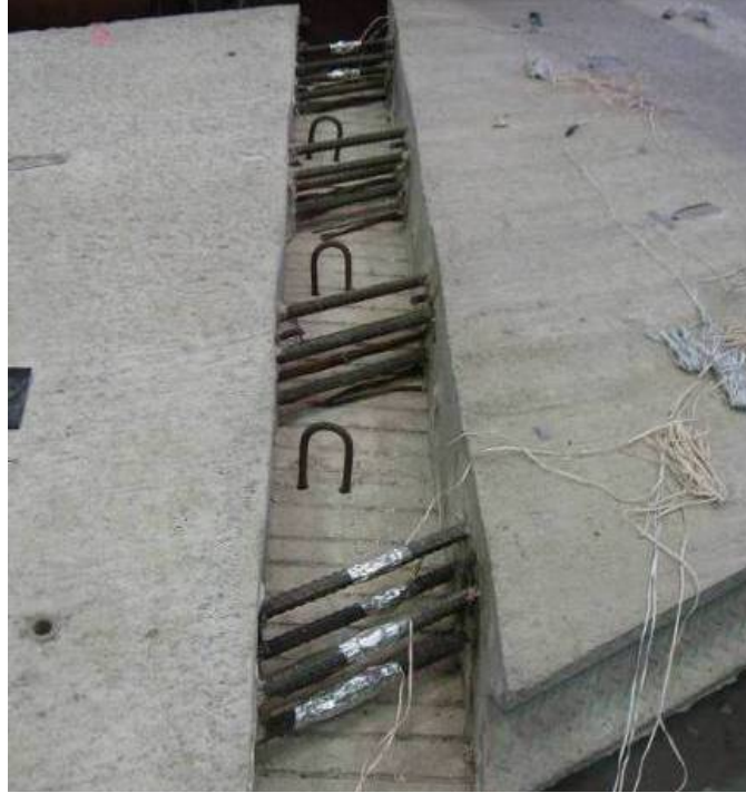
Figure 2.10. Reinforcing bars instrumented with steel strain gages.
