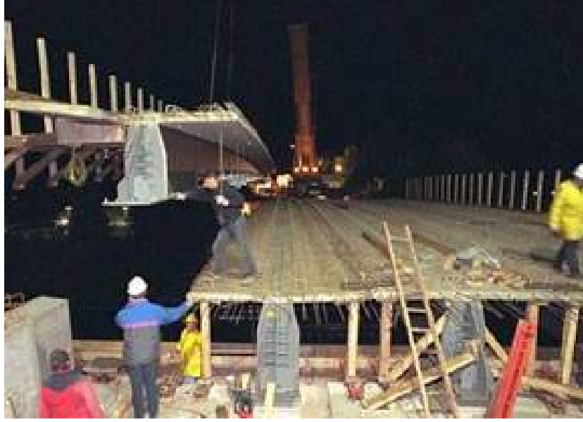
Figure 1.3. Placement of partial depth panels cast on beams (Russell et al. , 2005).
