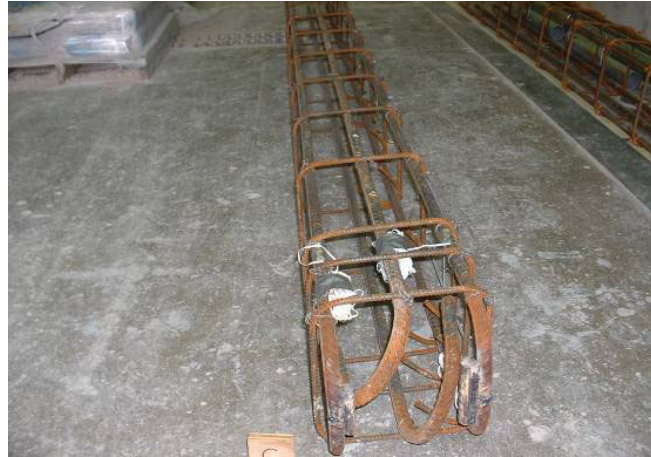
Figure 48. Photograph of Column 4, 12 ft. segment reinforcement.
