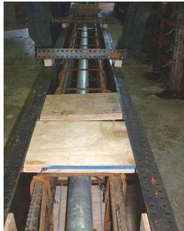
Figure 45. Photograph of Column 3 reinforcement and inserts.
