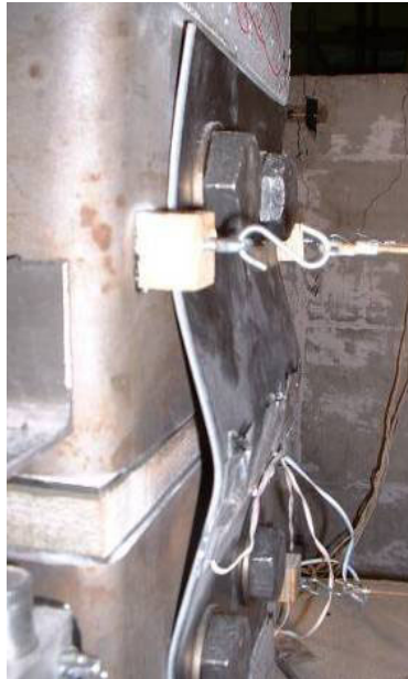
a.) West fuse plate buckling
