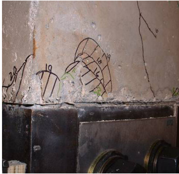
b.) Southeast corner interface opening
