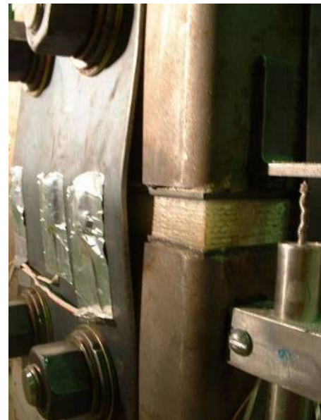
b.) East fuse plate buckling
