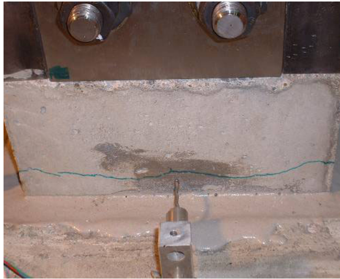
b.) East base initial cracking
