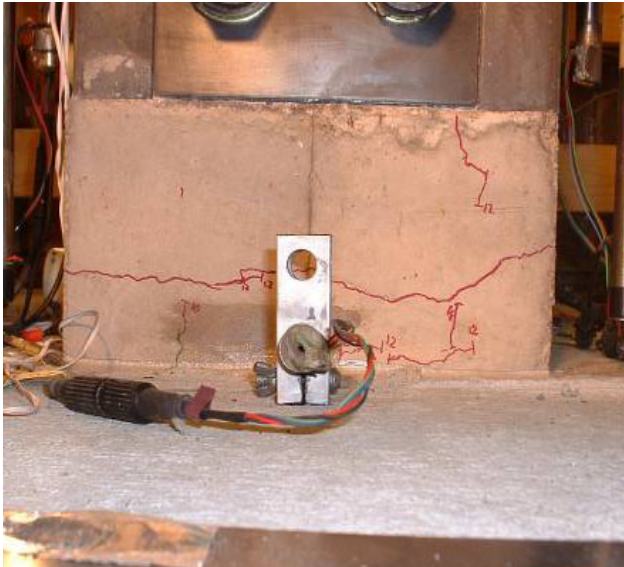
a.) East base cracking
