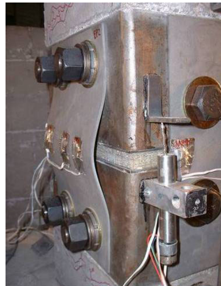
d.) West fuse plate buckling
