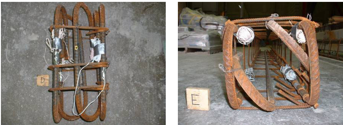
a.) Columns 2-4, 2 ft. segment reinforcement
