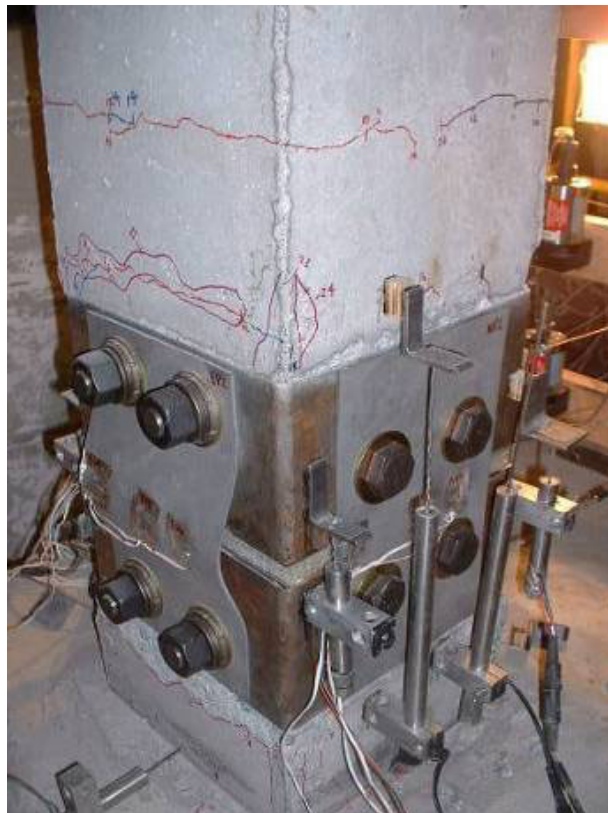
Figure 155. Photograph of Column 6 – Cycle 26b, column damage.
