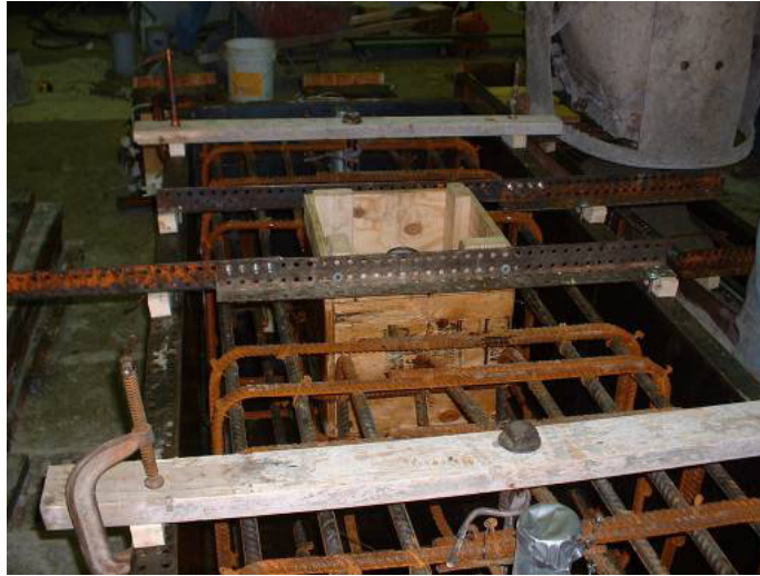
Figure 50. Photograph of Column 4 foundation reinforcement in forms.
