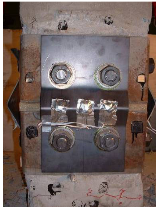
d.) South face after test
