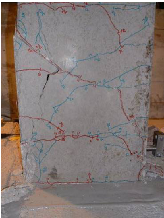
c.) North face cracking/spalling
