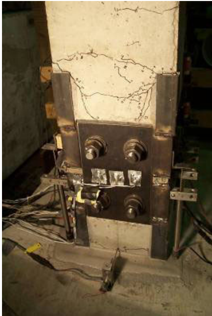
a.) East face crack progression
