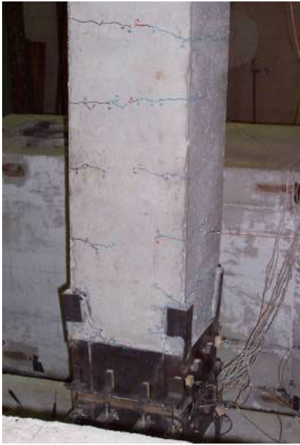
a.) Northwest corner damage
