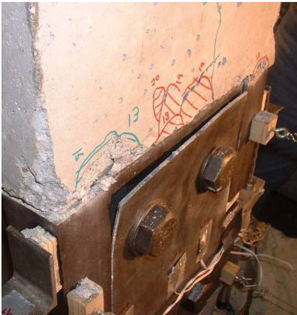
c.) West bolt bearing causing plate curling
