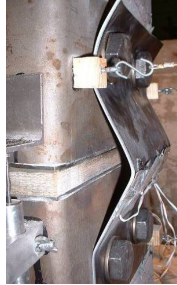
b.) West fuse plate buckling
