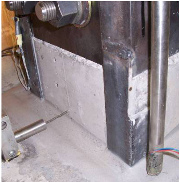
a.) Northwest retrofit angle on bottom column segment
