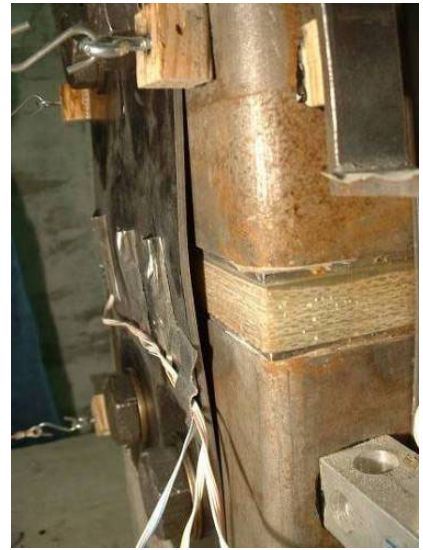
b.) West fuse plate initial buckling
