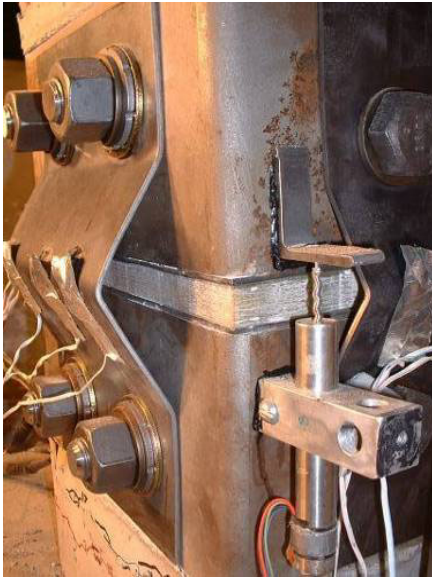
a.) East fuse plate buckling
