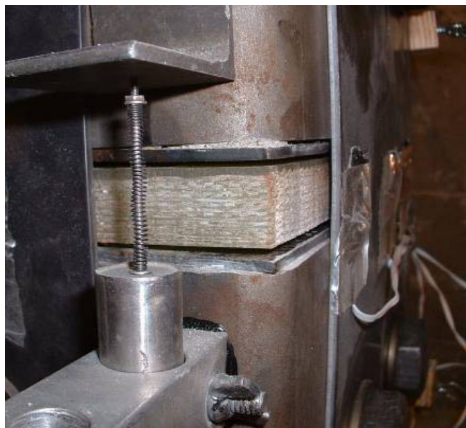
b.) West joint opening during pull half-cycle
