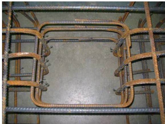
Figure 25. Photograph of center socket reinforcement.
