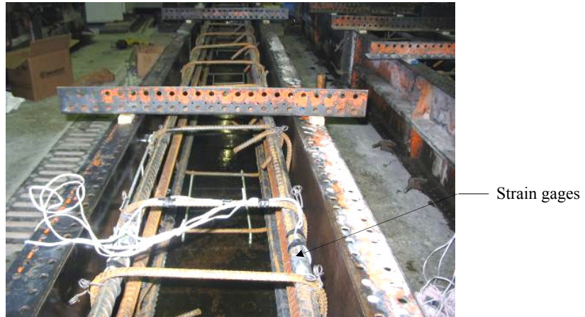
Figure 30. Photograph of Column 1 reinforcement.
