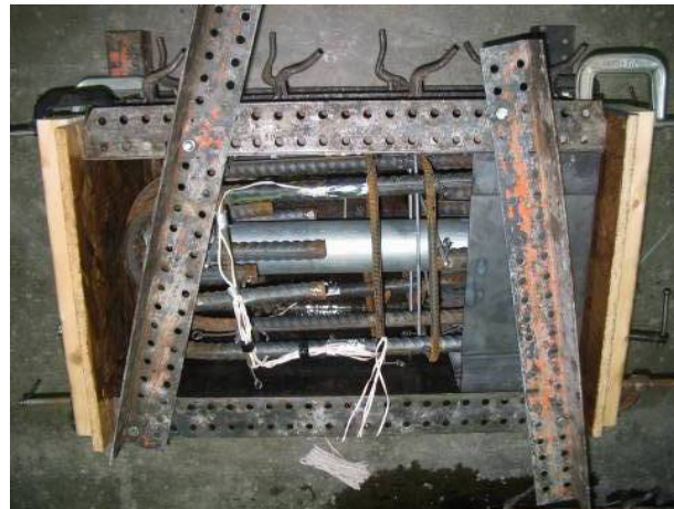
Figure 39. Photograph of Column 2 reinforcement in forms.
