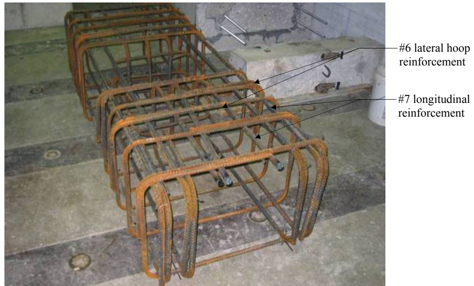
Figure 26. Photograph of foundation reinforcement cage.
