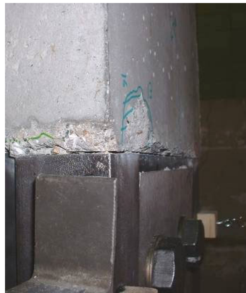
b.) Northwest corner interface opening
