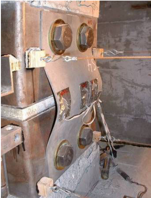
a.) West fuse plate buckling
