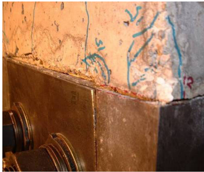
b.) Northeast corner collar/column interface
