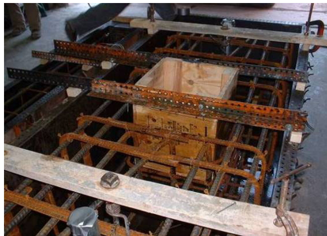
Figure 49. Photograph of Column 3 foundation reinforcement in forms.
