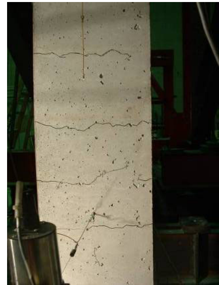
b.) Upper segment crack progression
