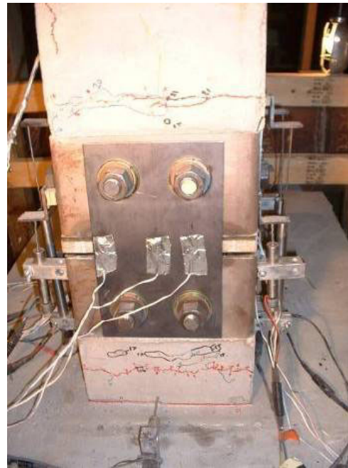
d.) East joint opening and segment damage
