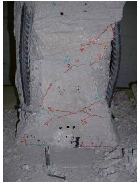
d.) Final damage to south face
