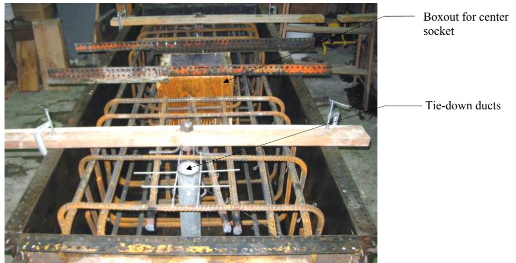
Figure 28. Photograph of foundation reinforcement and tie-down ducts in forms.
