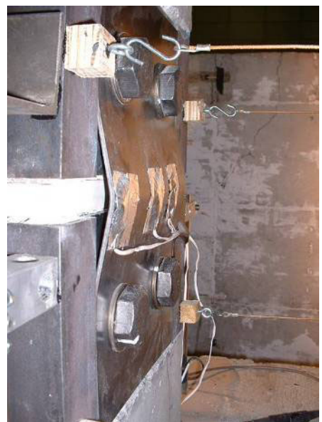
d.) Buckling of replaced west plate
