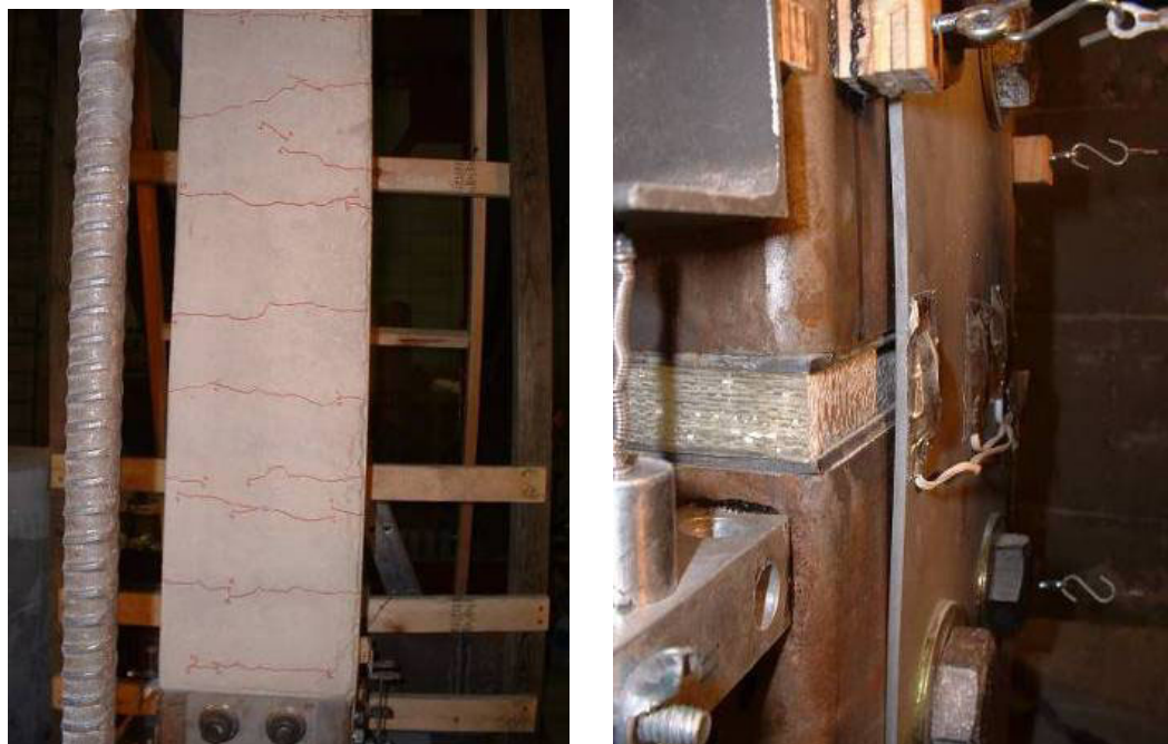
a.) East face of upper segment crack distribution
