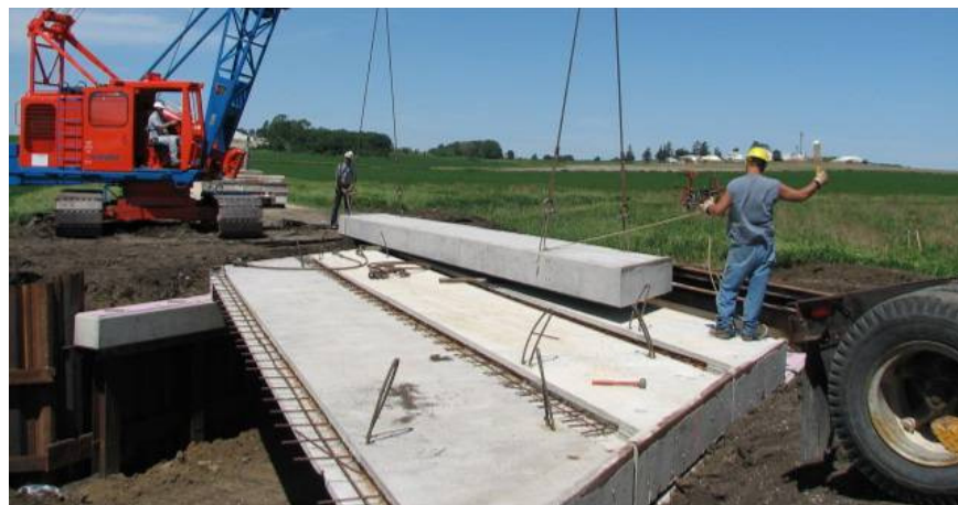
Figure 72. Setting panel on superstructure.
