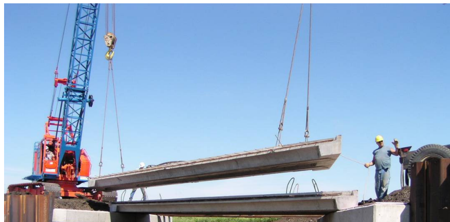
Figure 71. Using two cranes to position a deck panel.
