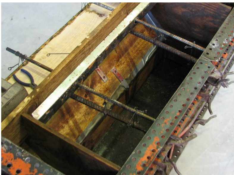
Figure 18. Photograph of reinforcement in forms.
