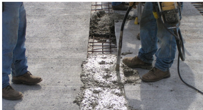
Figure 74. Closure concrete placement.
