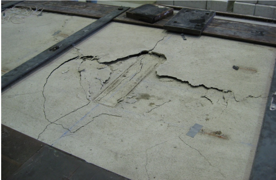
Figure 66. Failed abutment backwall specimen.
