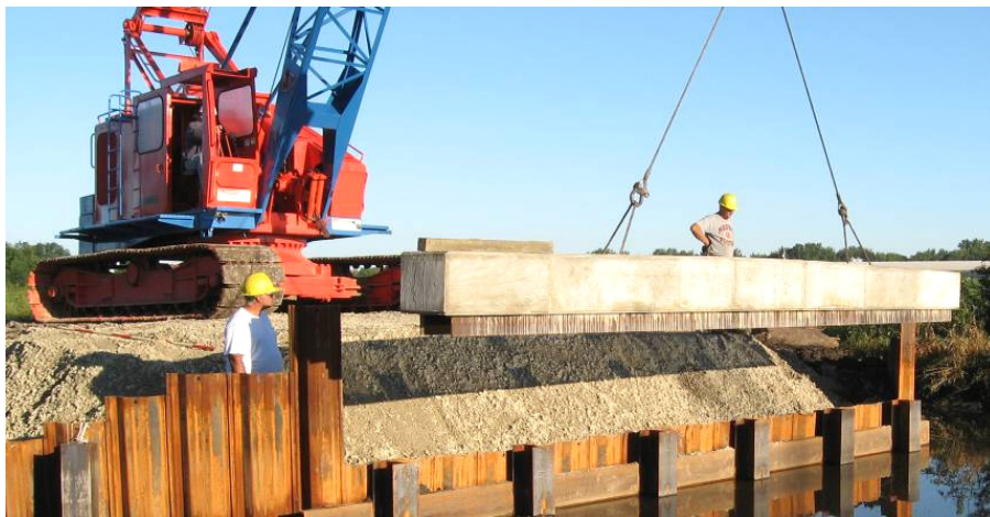
Figure 79. Placement of the precast abutment cap for the MRB.
