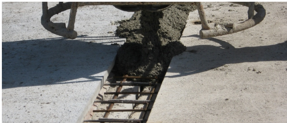
Figure 80. Using concrete bucket for placement.
