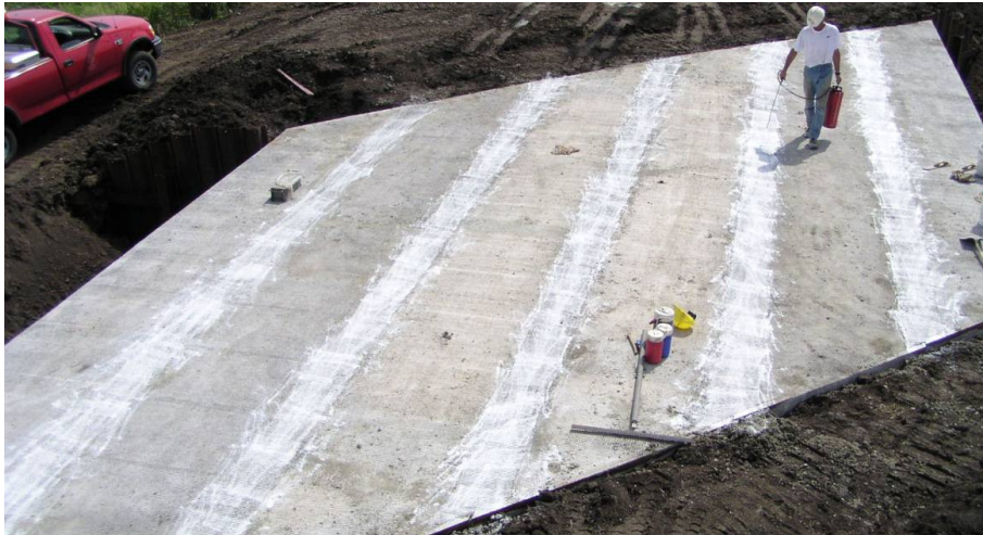
Figure 75. View of completed bridge.
