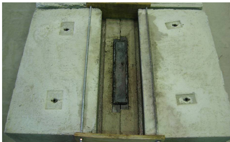
Figure 25. Type 2 Connection prepared for closure pour.
