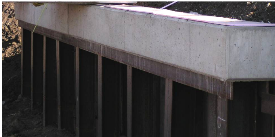
Figure 69. Abutment cap on H-piles.
