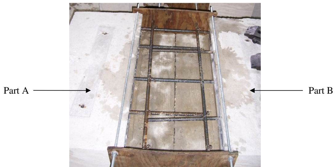
Figure 20. Position of reinforcing bar before closure.
