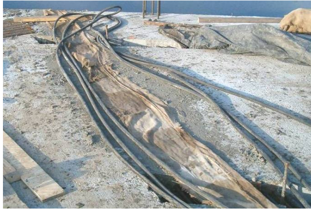
Figure 138. Burlap and heating coils on the west end panel joint, November 16.
