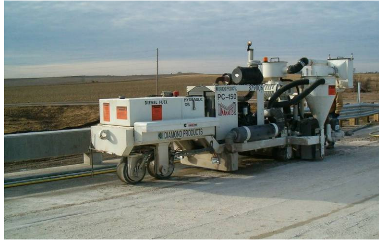
Figure 148. Bridge deck grinding equipment on site, December 27.
