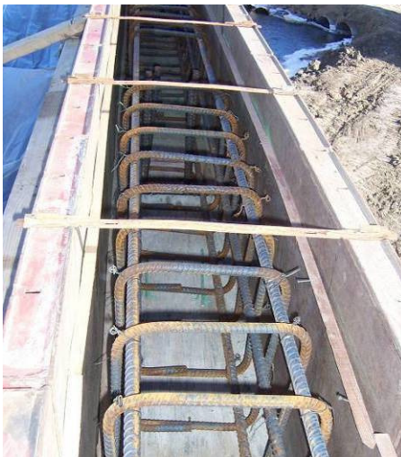
Figure 146. Barrier rail reinforcement, December 8.
