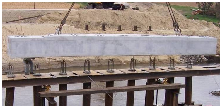
Figure 118. West pier cap being lowered into place, October 4.
