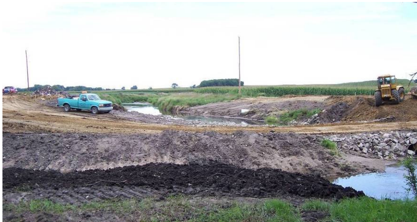
Figure 105. Cleared bridge site, August 7.
