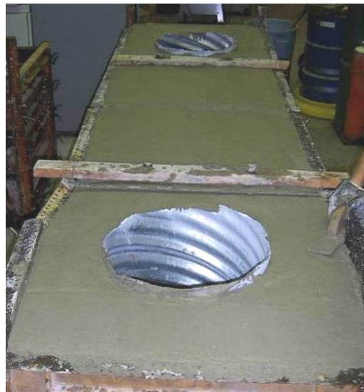
Figure 33. Abutment 6 after hand-finishing.
