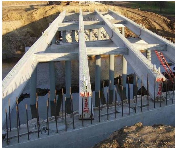
Figure 128. Erected bridge girders, October 24.
