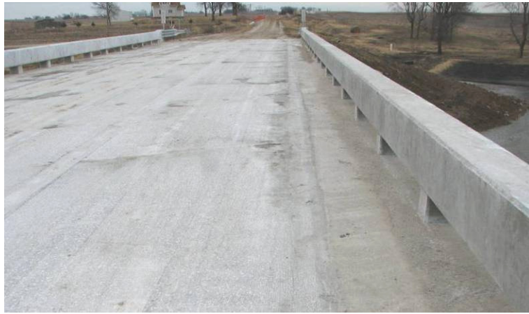
Figure 149. Bridge deck after the surface was ground, December 27.
