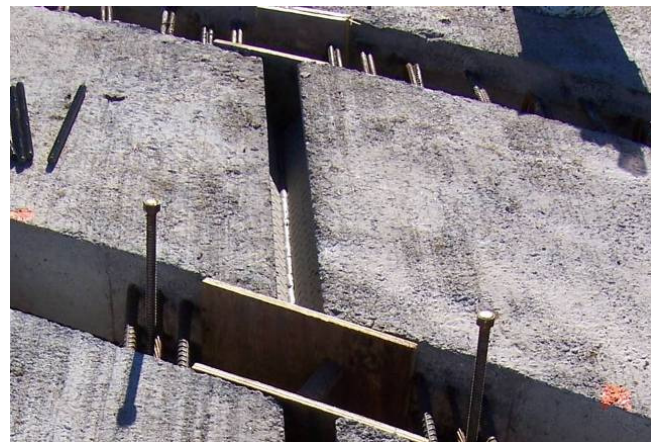
Figure 133. Transverse joint formwork, November 5.
