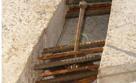
Figure 130. Deck panel leveling screw, October 26.
