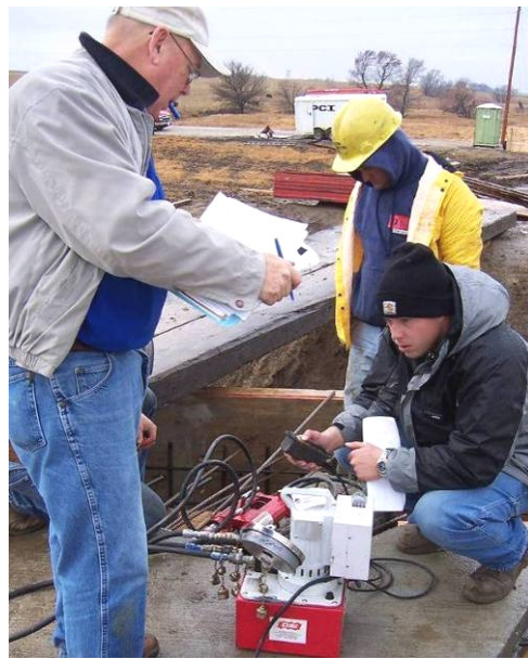
Figure 140. Post-tensioning in progress, November 28.
