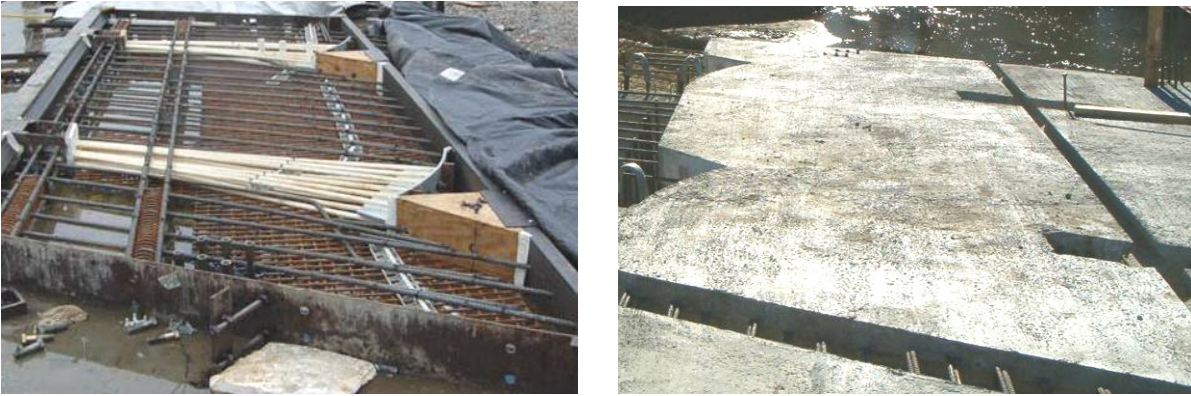
a) end panel reinforcement
