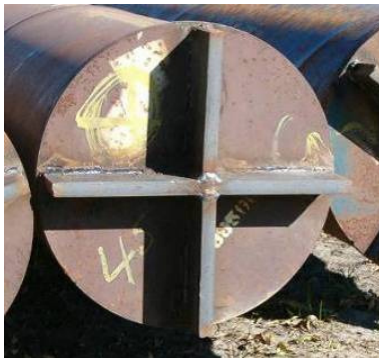
Figure 113. Steel pipe pile driving point, September 28.
