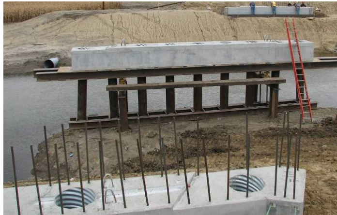
Figure 120. Precast abutments and pier cap in place, October 4.
