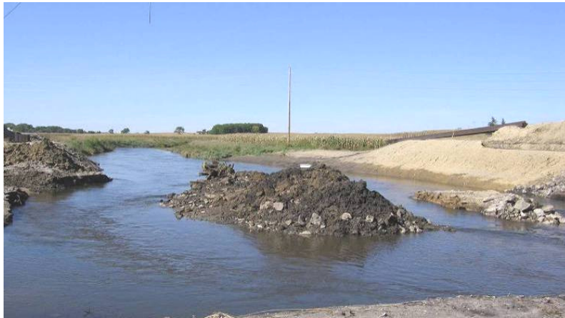
Figure 110. Bridge site on September 20.
