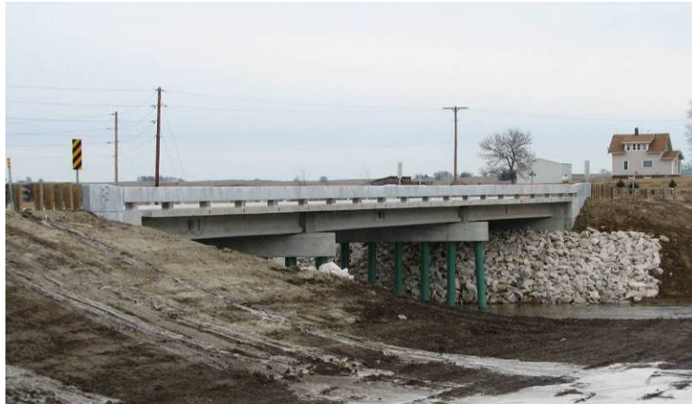
Figure 151. Completed bridge, December 27.
