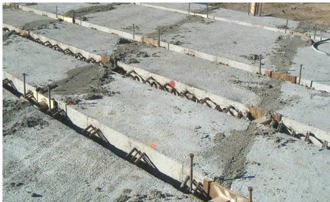
Figure 135. Several transverse joints before finishing, November 8.
