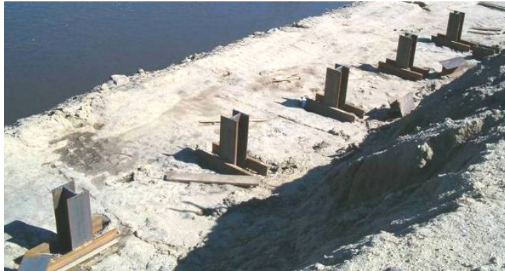
Figure 112. West abutment piles after wood blocking was removed, September 20.
