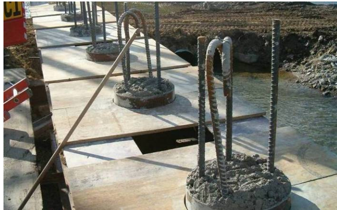
Figure 124. East pier pipe piles filled with concrete, October 12.
