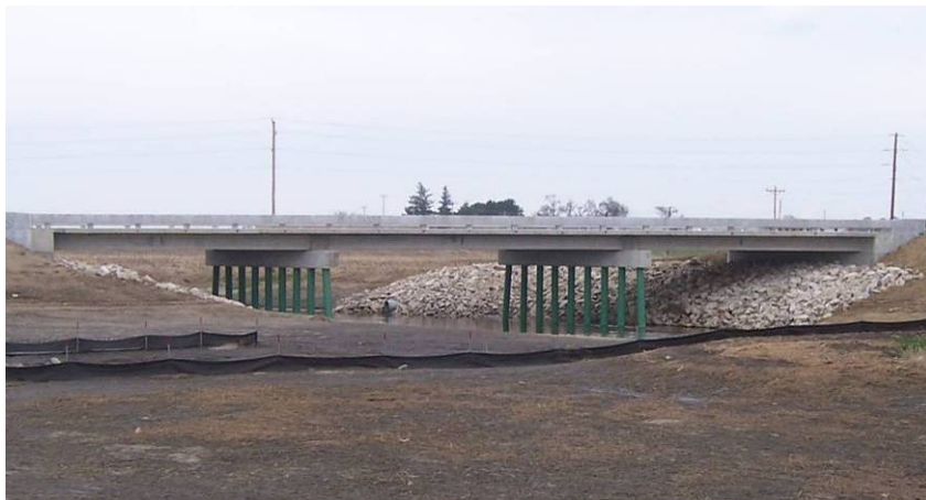
Figure 2. Completed replacement bridge on 120 th Street.
