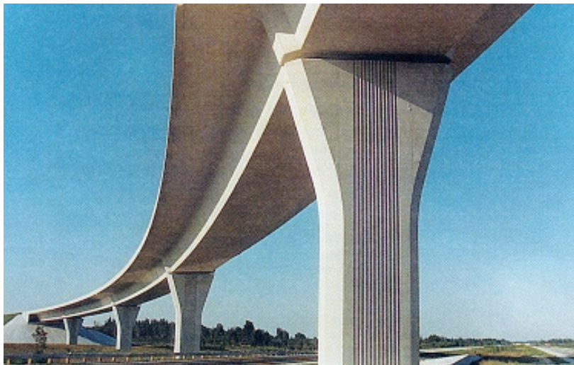
Figure 9. Slender pier design of the Florida Turnpike in Miami, Florida.
