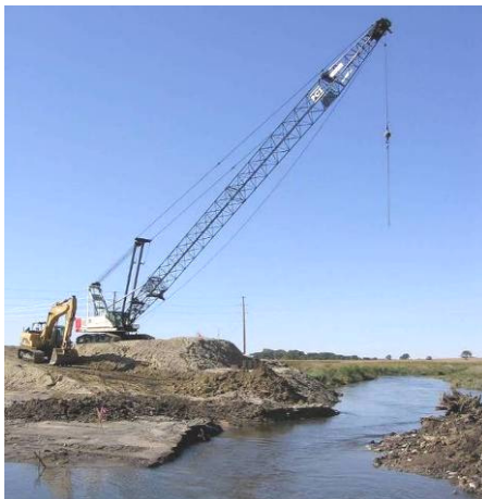
Figure 111. Damage to the west bank caused by the rain, September 20.
