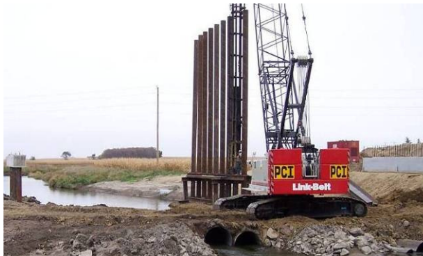
Figure 123. East pier pipe piles being driven, October 10.
