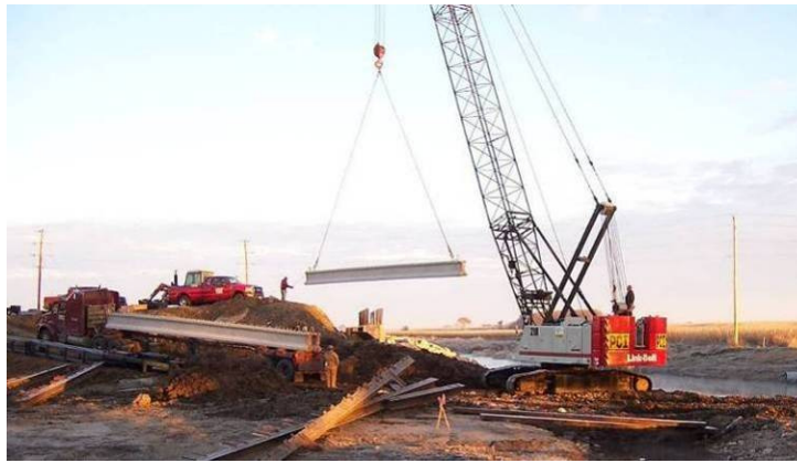
Figure 126. The first bridge girder being lifted into place, October 24.
