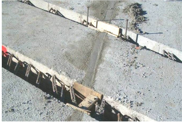
Figure 136. Finished transverse joint, November 8.
