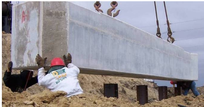
Figure 116. West abutment being lowered in place, October 4.
