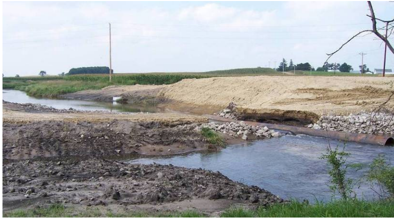
Figure 106. Access road and bridge site, August 11.
