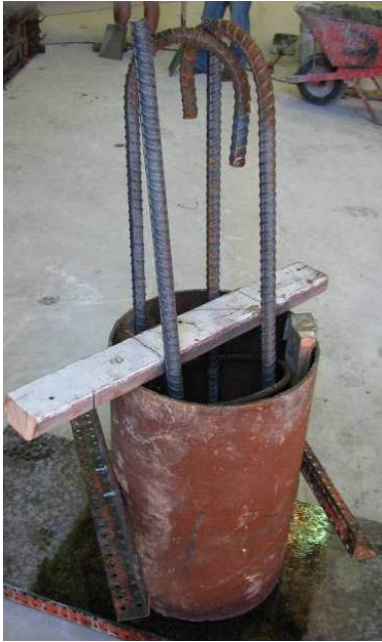
a) pipe pile before placing concrete
