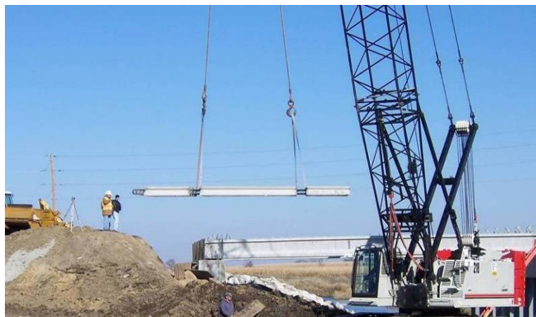
Figure 129. Deck panel being reset on the bridge girders, October 25.
