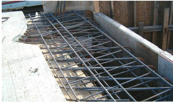
Figure 143. Reinforcement in the west abutment cap, November 29.
