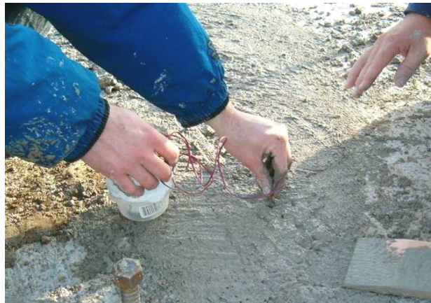
Figure 137. Thermal couple being inserted into end panel joint, November 16.
