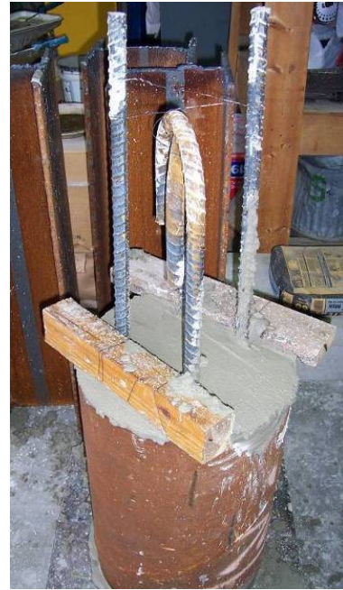
b) pipe pile after placing concrete
