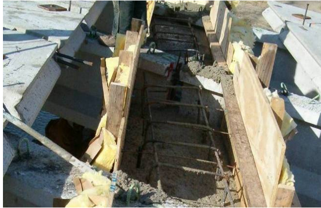
Figure 131. Pier diaphragm before concrete placement was complete, November 3.
