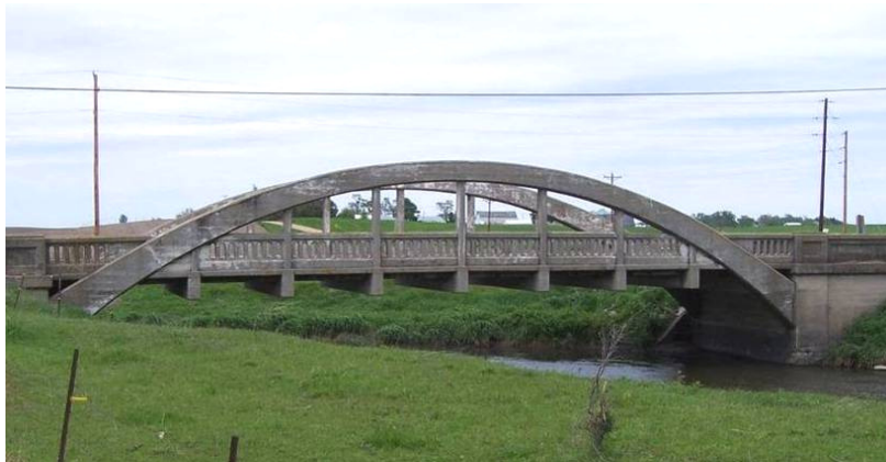
Figure 102. Previous bridge on 120 th Street, July 19.
