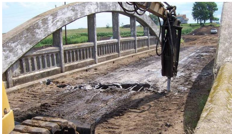
Figure 104. Breaking apart the Marsh Arch bridge deck with a back hoe, July 24.
