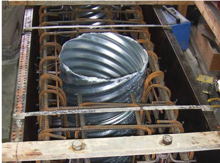
Figure 27. Pier cap reinforcement.
