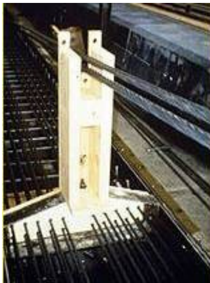
Figure 3. Bulkhead in a prestressed concrete casting bed.
