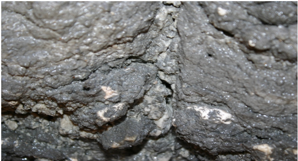
Figure 5.12. Slurry encased in void in 90 sec/qt shaft.
