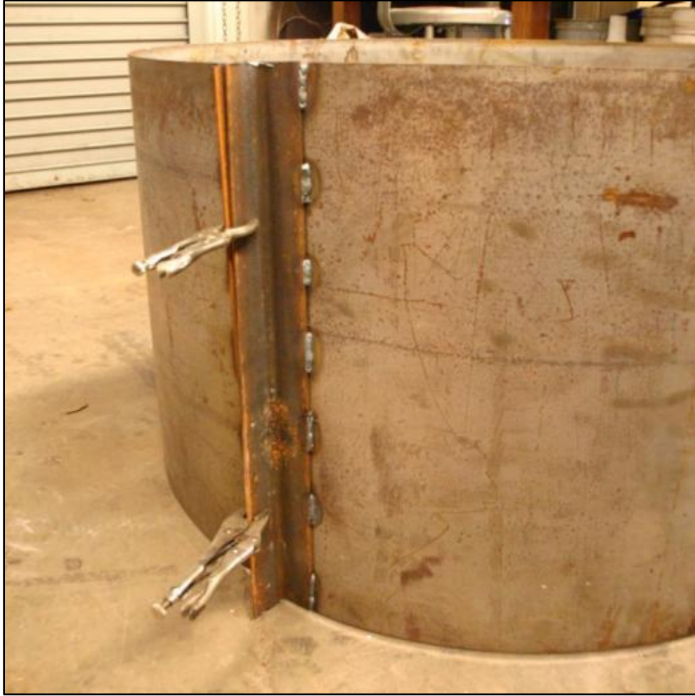
Figure A.3. Steel form, clamped, welded angle closures.
