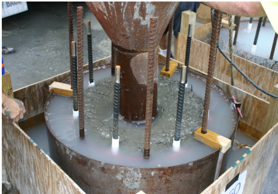
Figure 3.13. Placing concrete via tremie.
