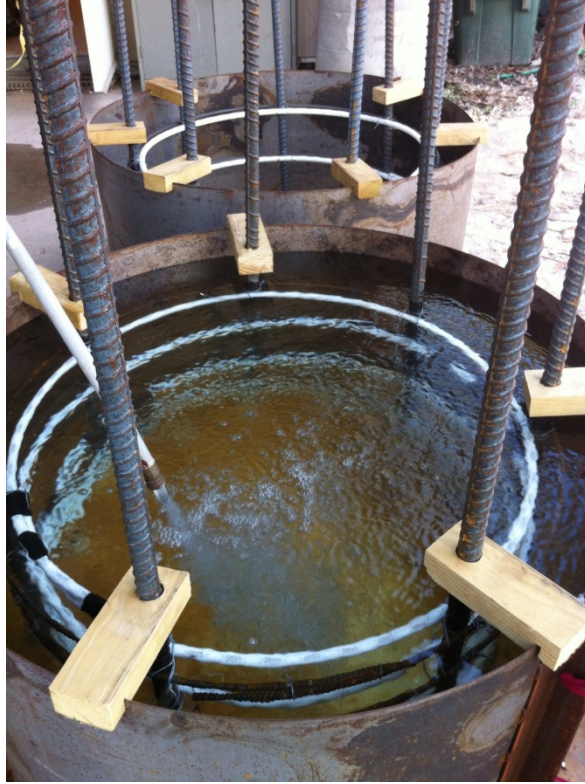
Figure A.8. Verifying water tight seal of form.
