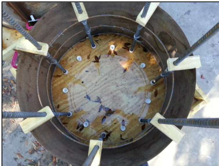
Figure A.5. Form with structural reinforcement prior to placement of pullout steel.
