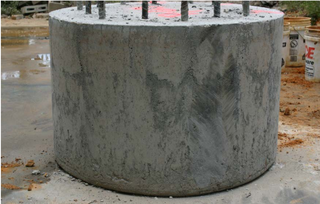
Figure 4.12. Shaft cast with polymer slurry following pressure washing.
