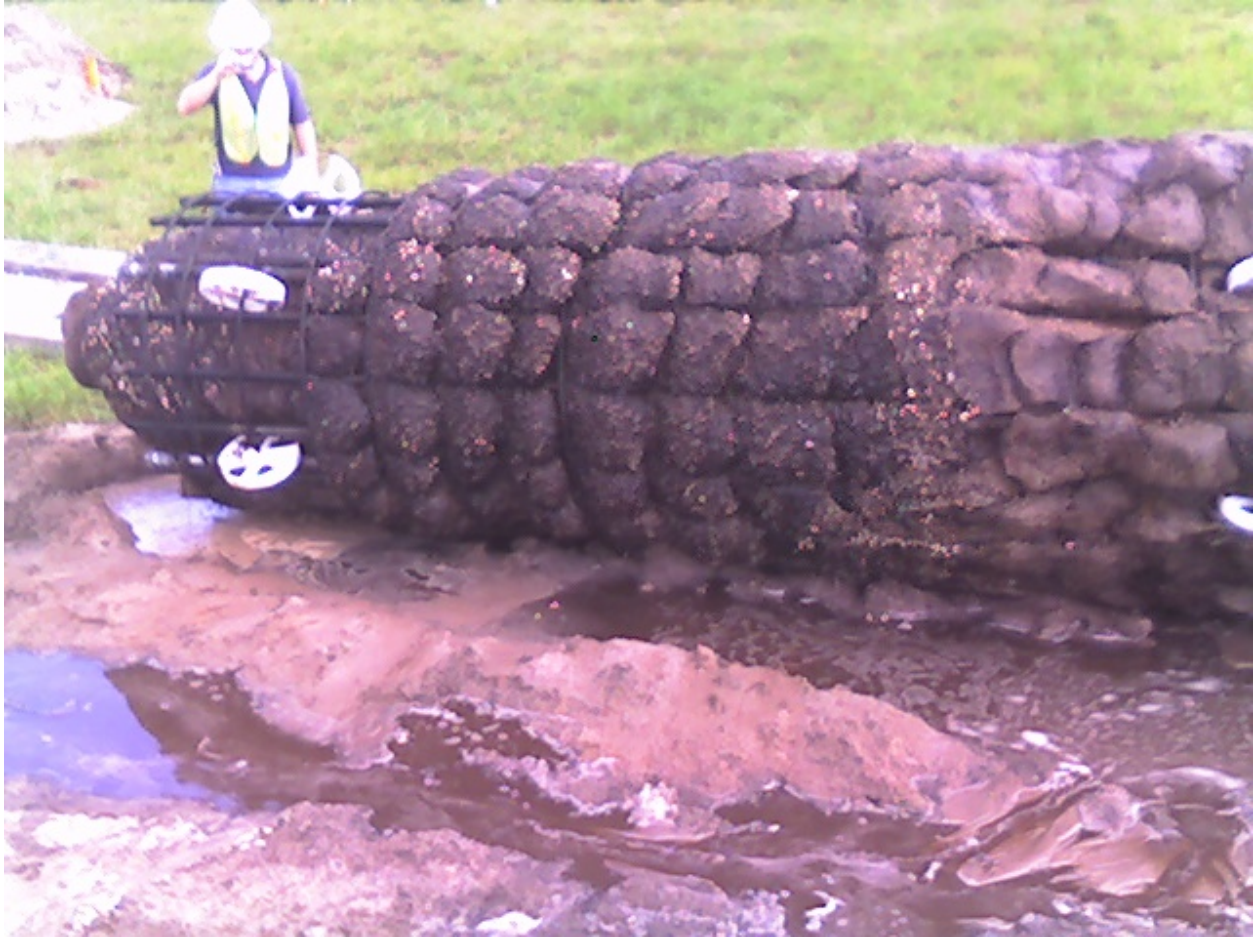
Figure 2.9. Exhumed drilled shaft displaying concrete flow issues.
