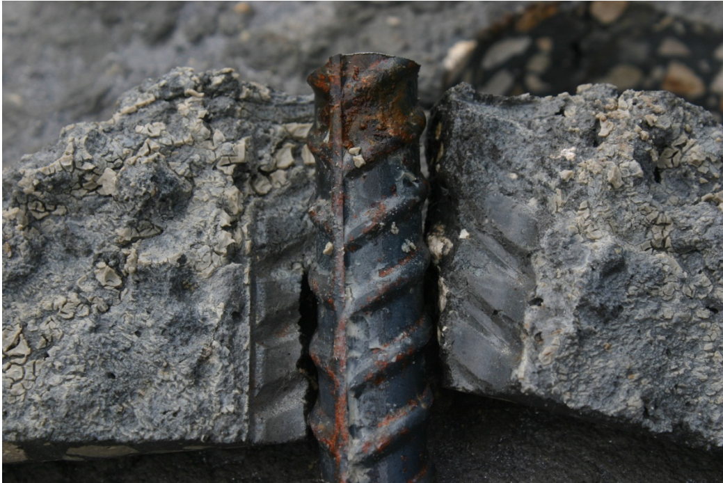
Figure 5.6. Layer of slurry encased in concrete.
