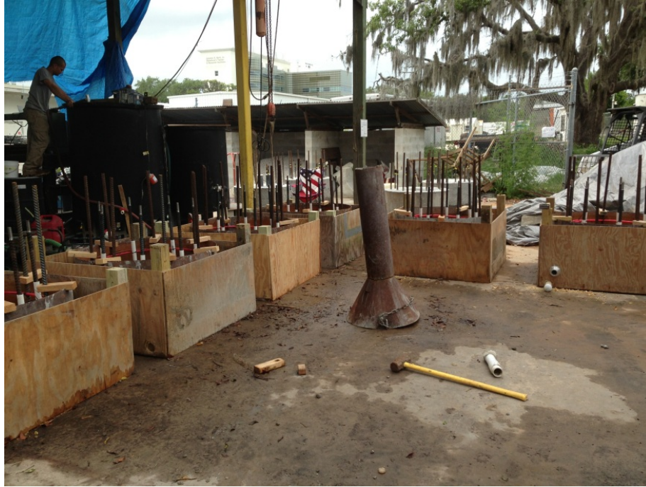
Figure A.14. Form layout for placements 2 through 4.
