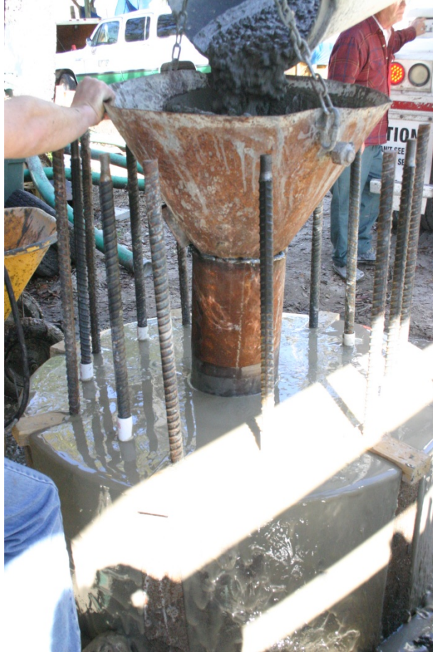
Figure A.12. Placing concrete for shaft 1, 40 sec/qt mineral slurry.
