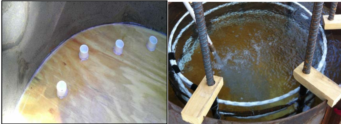
Figure 3.5. Silicon to seal form (left), water testing to ensure water tight seal (right).
