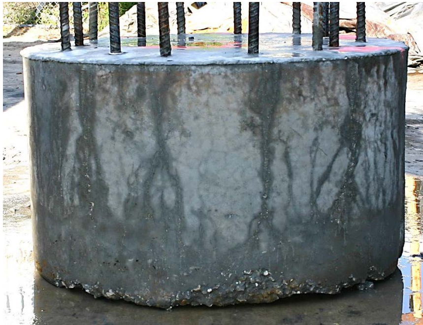
Figure A.15. Shaft 6 (water) after pressure washing.
