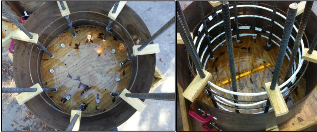
Figure 3.6. Structural, outer layer, reinforcement (left) and full cage (right).
