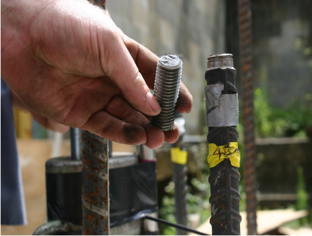
Figure A.34. Bar failure from shaft 6, water.
