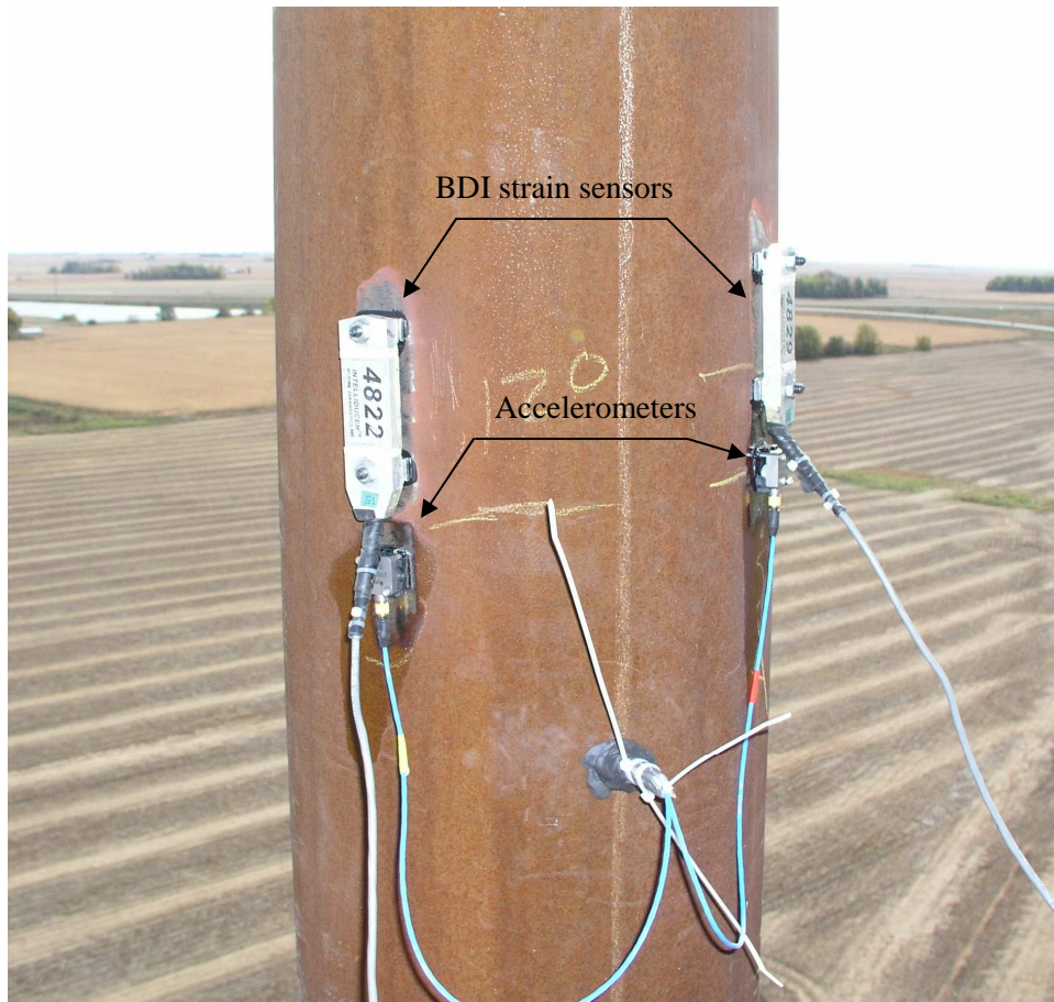
Figure 3-9. Temporary BDI gages and accelerometers on Pole 1
