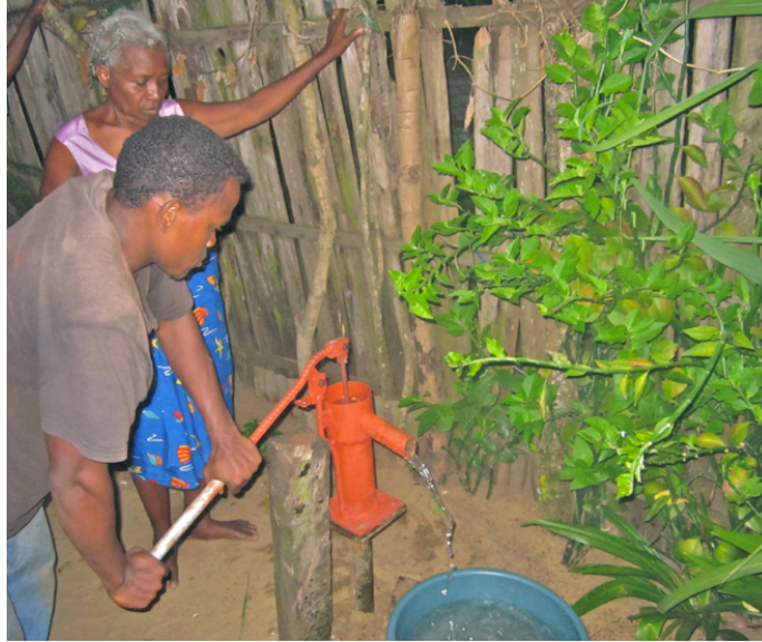
Figure 11. Finished retrofitted pump with pump manufacturer (pumping) and owner (behind).
