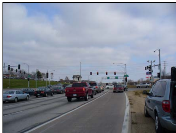
Figure 103. Kimberly & Elmore Ave. (eastbound).
