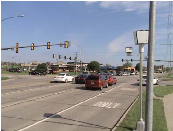
Figure 32. 100th St. & Hickman Rd. (northbound).
