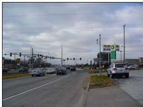
Figure 93. Kimberly Rd. & Brady St. (westbound).
