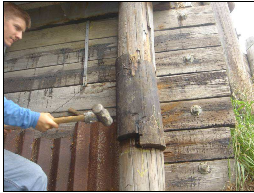
FIG. 5.10 — Repairing pile No. 7 using the splicing technique
