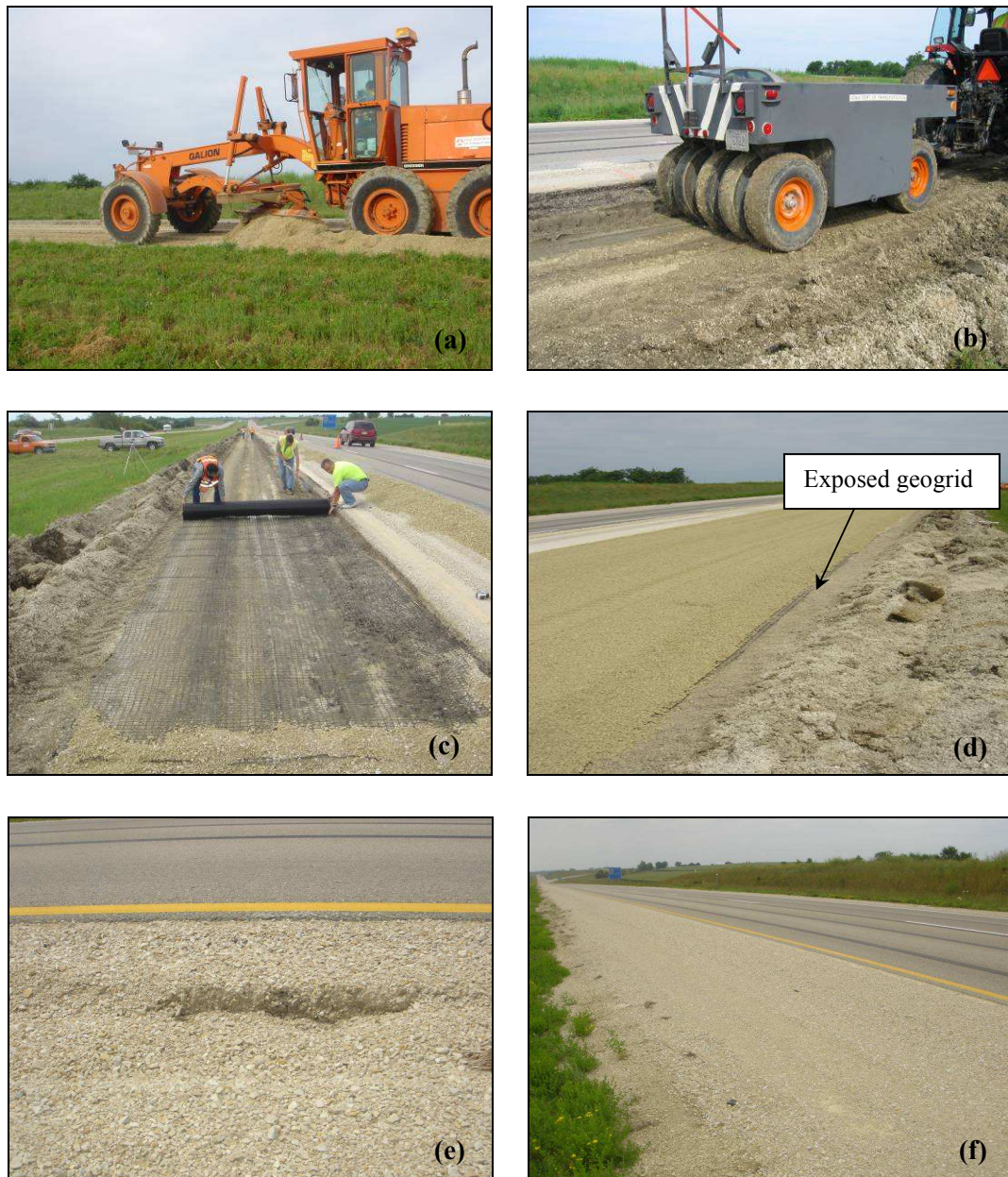
FIG. 3.5 — Shoulder reconstruction using geogrids (a) motor grader removing the contaminated granular layer (b) pneumatic roller used to compact the subgrade (c) rolling the geogrid over the subgrade (d) spreading the aggregate over the geogrid (e) rutting developed at the control section after one month (f) no rutting at the geogrid stabilized section after one month
