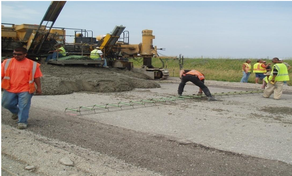
Figure 4.14 Overlay Pavement Construction
