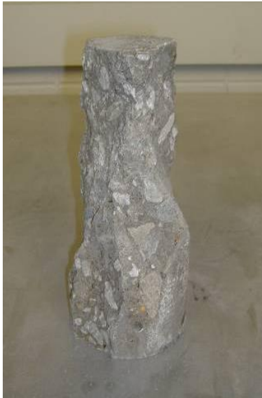
Figure 4.12 Visual Segregation Inspection
