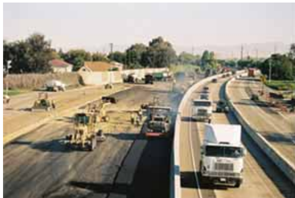
Figure 13. Caltrans I-710 Full Closure (94)
