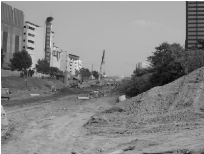
Figure 14. M-10 Lodge Freeway, Detroit, Michigan (95)
