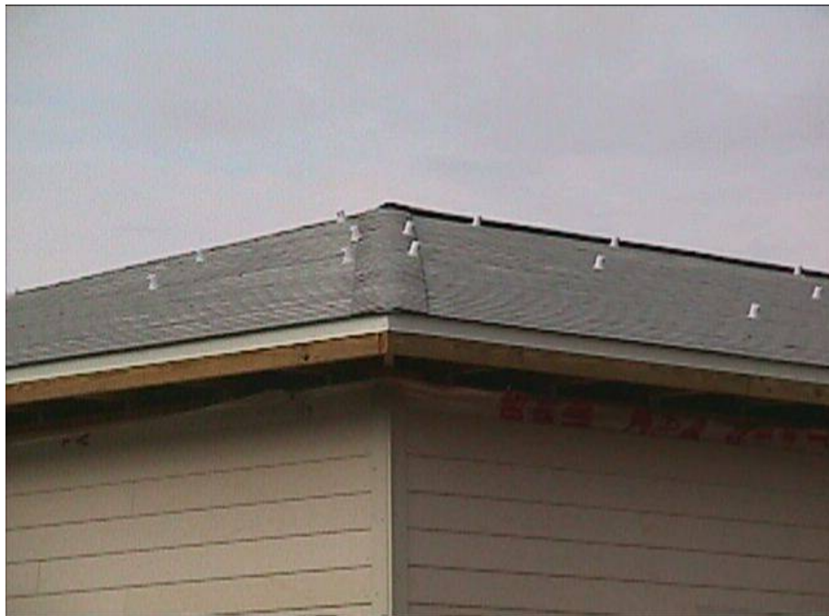
Figure 3.10. A view showing the pressure ports on the hip roof (FPL, 2006)
