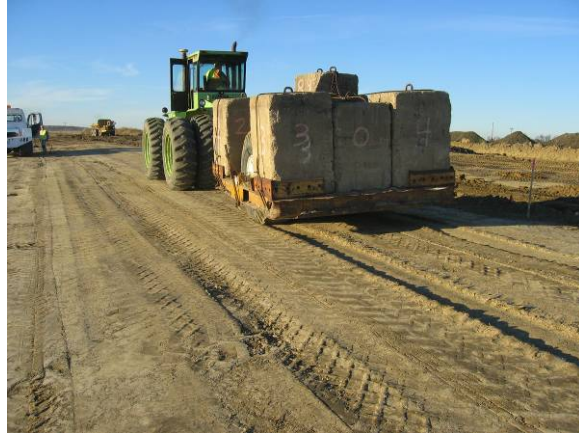
Figure 2.12. Test roller and subgrade rutting observed following test rolling
