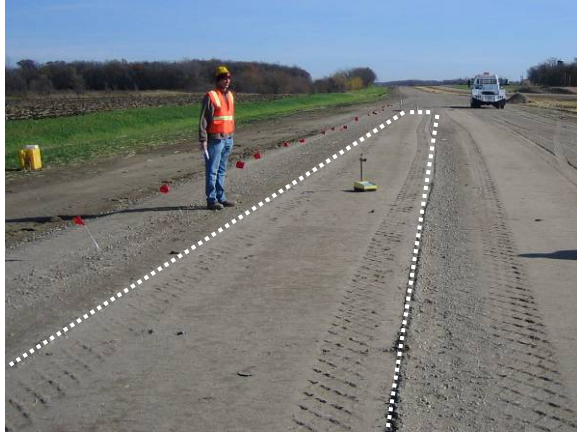
Figure 2.9. Test strip comprised of Class 5 material (outlined with dashed line) for evaluating variable feedback control operation
