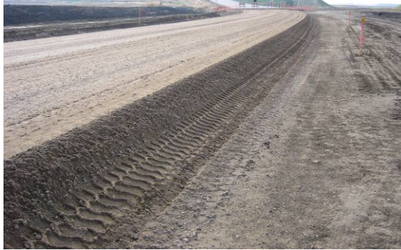
Figure 6.1. Strip 1, comprised of Class 5 subbase material overlying compacted subgrade
