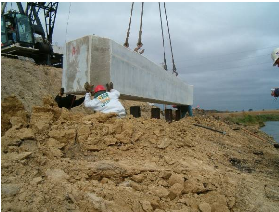
Figure 5. Setting precast abutment
