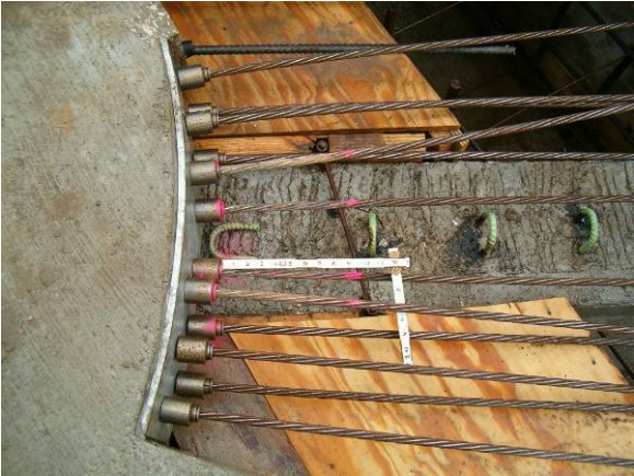
Figure 9. Strand elongation check
