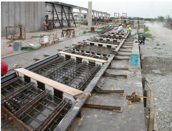
Figure 1. Panel forms and reinforcing
