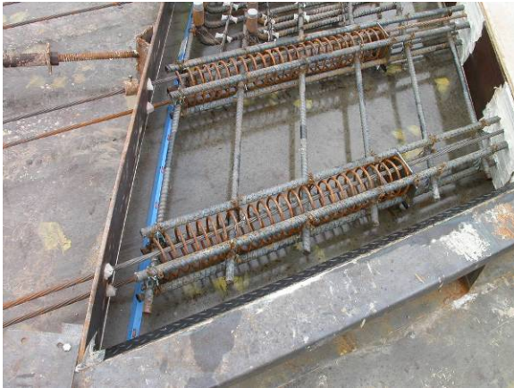
Figure 3. Spiral reinforcing
