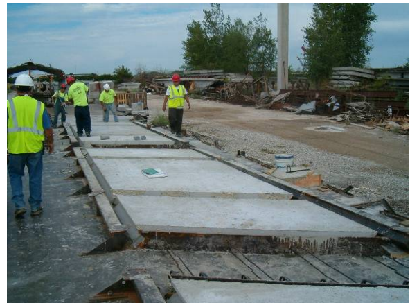
Figure 2. Panel form release
