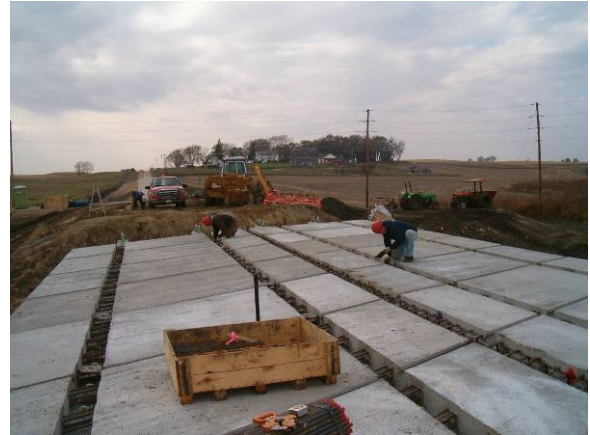
Figure 8. Leveling device installation
