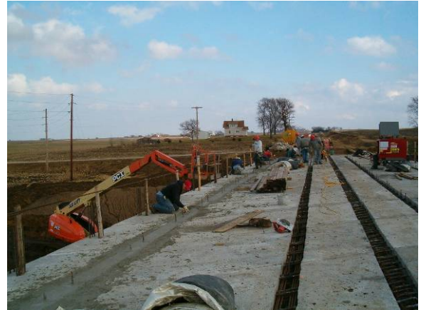
Figure 10. Casting longitudinal joints
