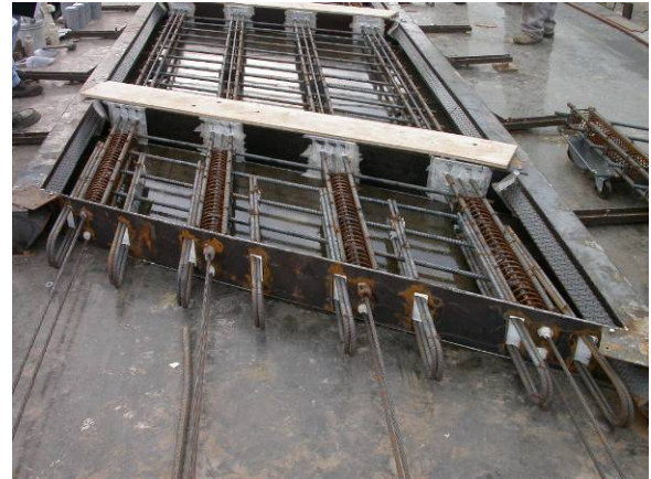
Figure 4. Longitudinal joint reinforcing
