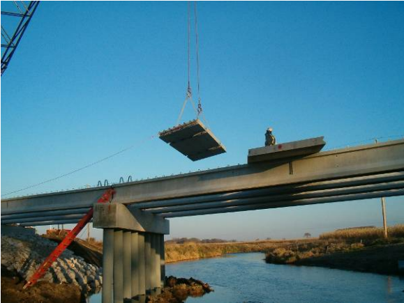
Figure 7. Deck panel erection
