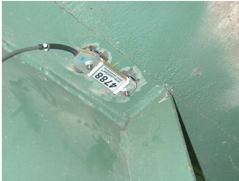
Figure 4.2. A BDI Intelliducer in use on a steel girder.
