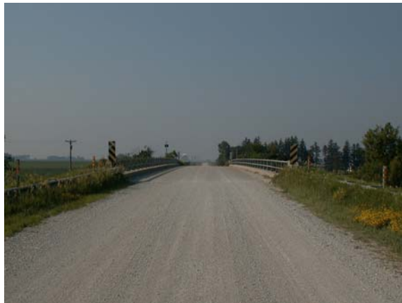
b. Photograph showing the roadway, deck, and railing of Bridge #2.
