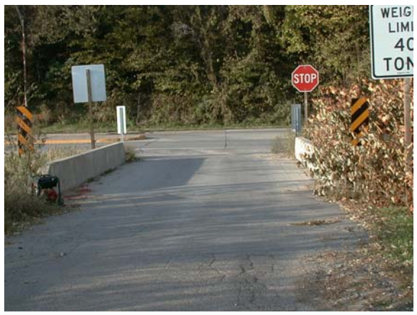
Figure 2.8. Roadway view of Bridge #3.
