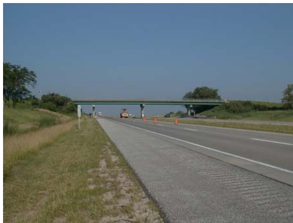
a. Photograph showing profile of Bridge #2 over I-80 in Iowa County.
