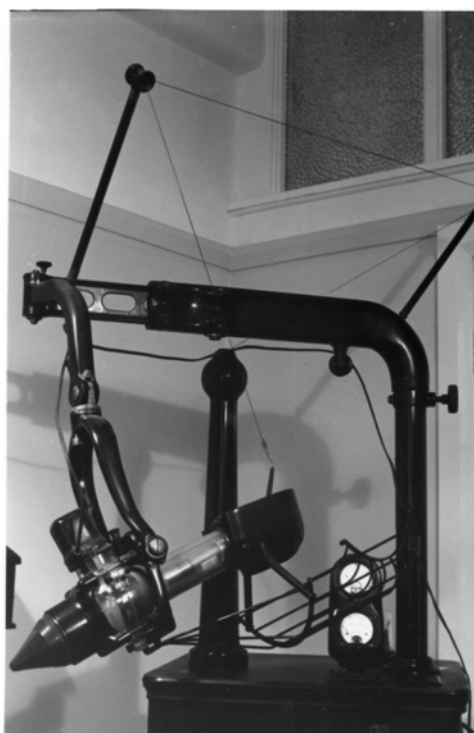
Figure 3.6: The Electrical Wiring (X-Ray) Regulations aimed to protect operators and patients from the electrical hazards associated with X-ray equipment. This dental X-ray machine, installed in the 1930s, had an uninsulated overhead high tension wire, which could have caused electric shocks if touched while in use. Source: National Radiation Laboratory, Christchurch, NZ.
