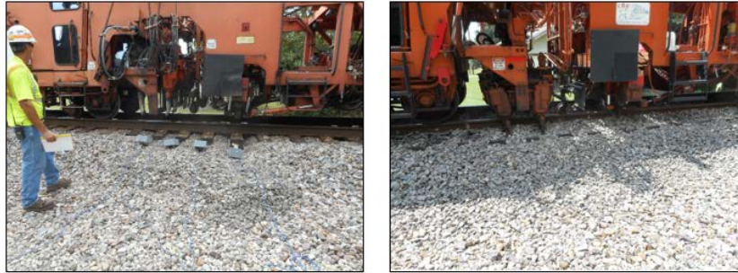
Figure 6.3 Tamping the Test Section
