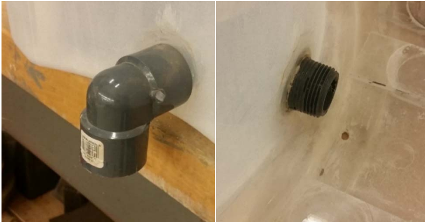
Figure 3.8: Outer (left) and inside (right) view of threaded elbow PVC connection to plastic container.
