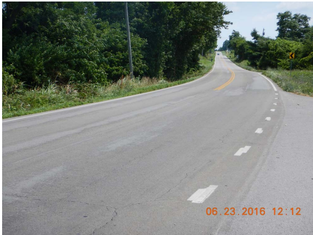
Figure 7.12: Boyle County, Surface Wearing, Microsurfacing
