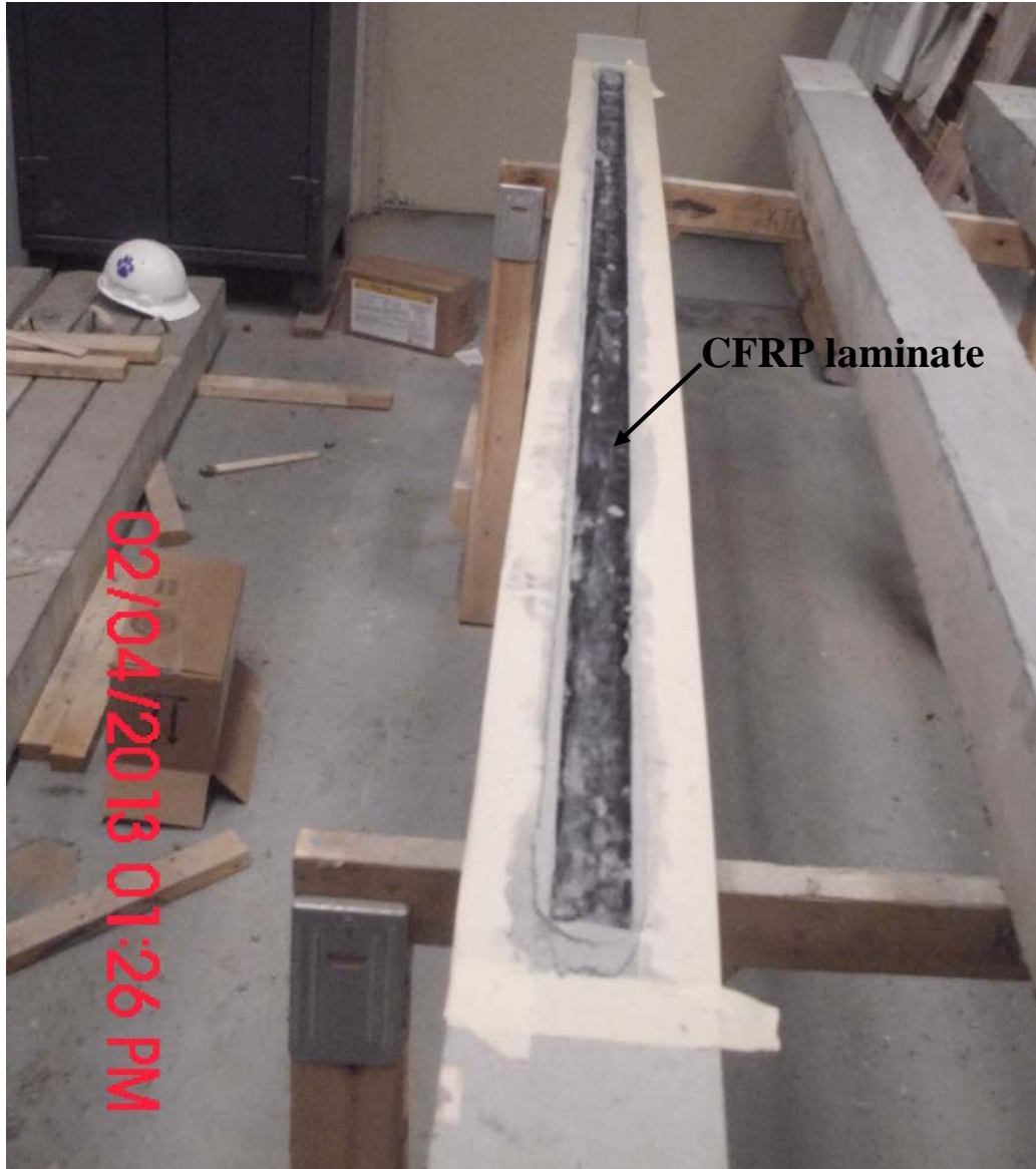
Figure 4.5 Installation of CFRP laminate.
