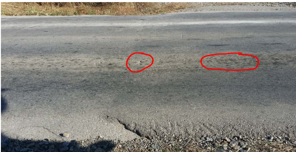
Figure 7.22 Crossing scratch marks A.
