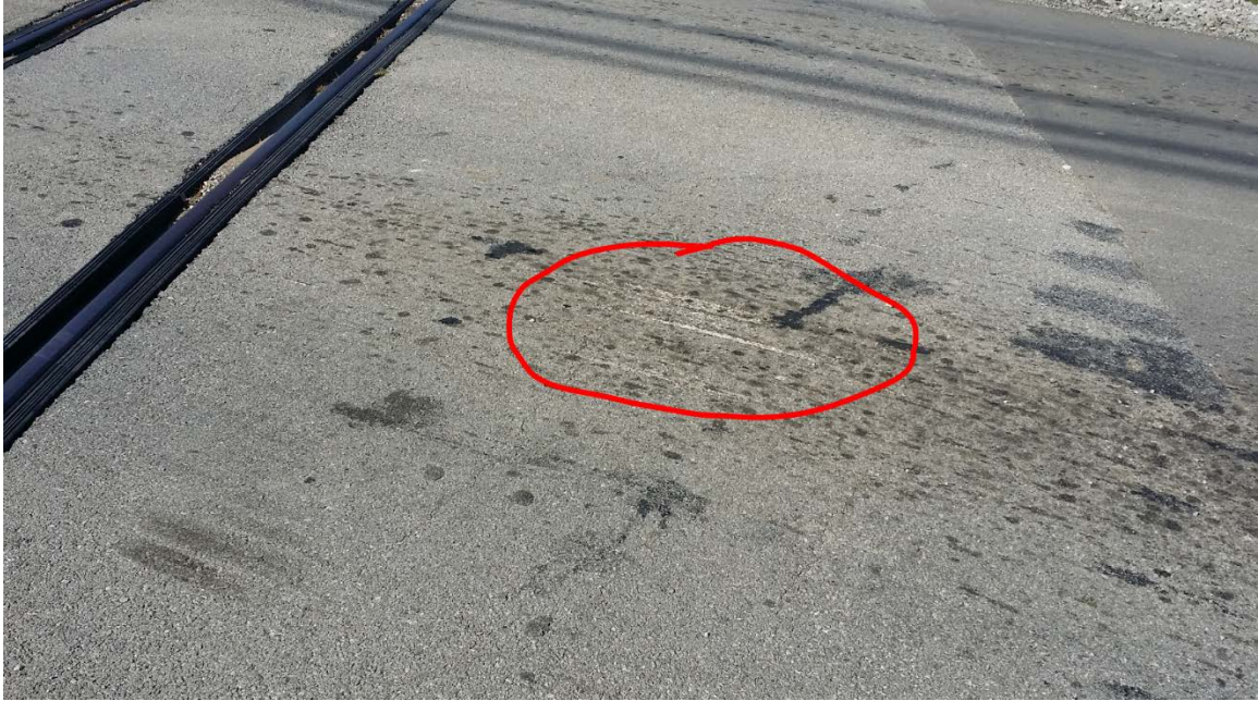
Figure 7.23 Crossing scratch marks B.
