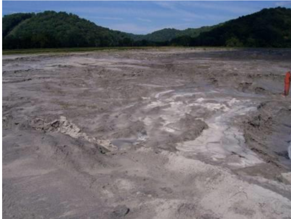
Figure 1.12: Fly ash impoundment at the DPL Power Plant after an accident
