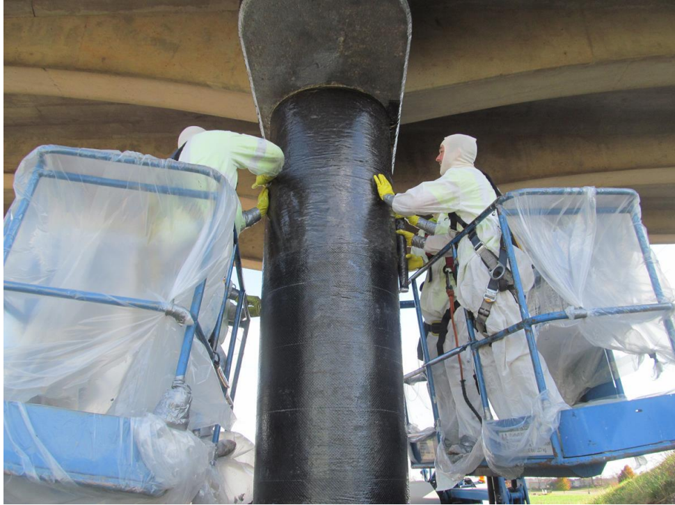
Figure 5.19 –Application of Triaxial Carbon Fabric
