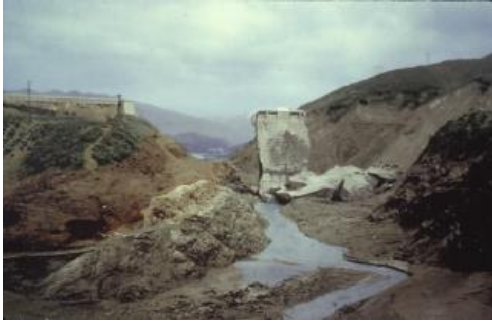
Figure 1.8 A picture of the damaged St. Francis dam in Los Angeles, 1928 (Rogers, 2007)
