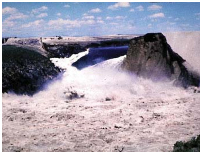
Figure 2.1: Teton Earthen Dam Failure in 1976 (Arthur, 1977).
